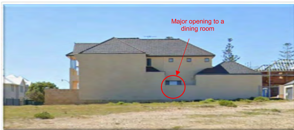
Figure 3: View of 23 Shoreham Turn
