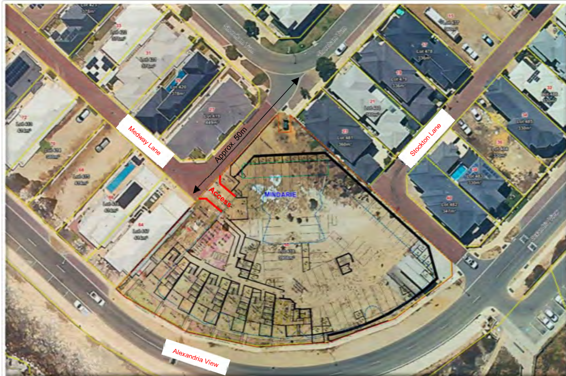
Figure 4: View of access location on Medway Lane
