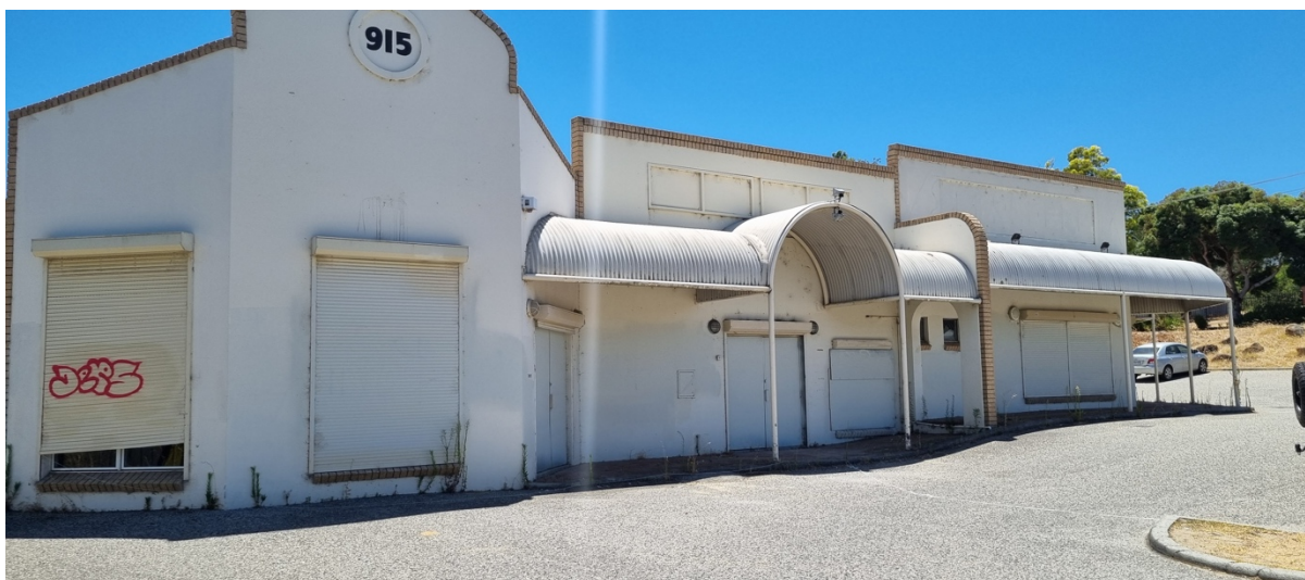
Photograph 1: The southern façade of the existing building.
