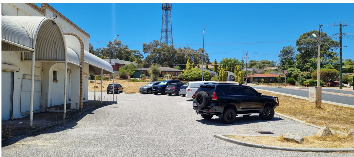
Photograph 3: Existing building, driveway and car park, looking east.
