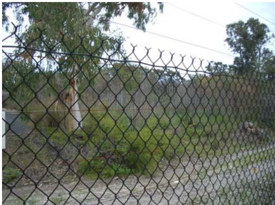
Plate 4.4 Cyclone fencing
