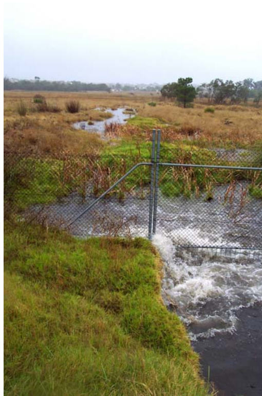
Figure 12a. In times of high flow rates after heavy rainfall, the untreated water from the Wangara Industrial area overflows directly into Walluburnup Swamp (Photos by John Chester taken in May, 2004).
