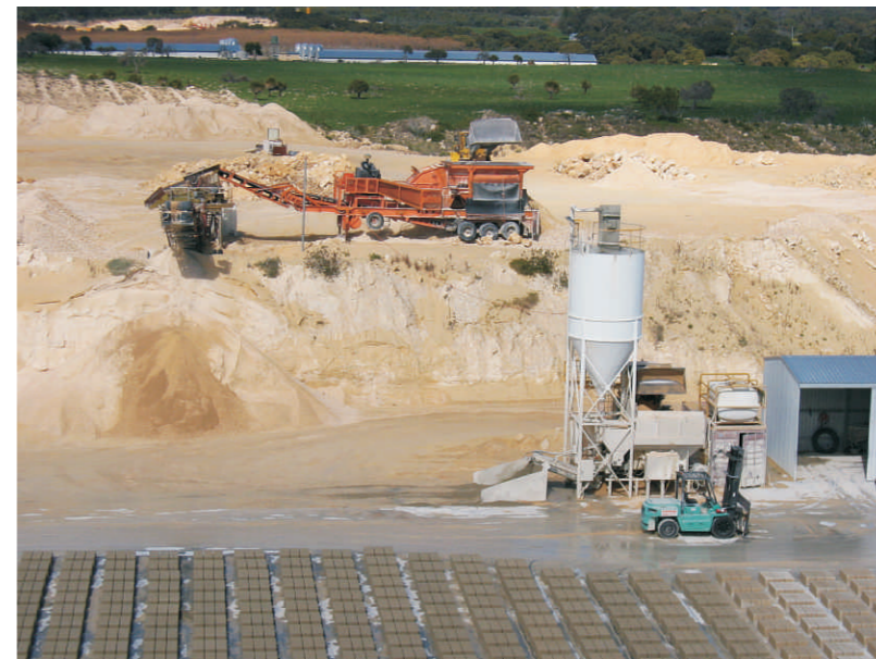
Mobile crusher and batching plant
