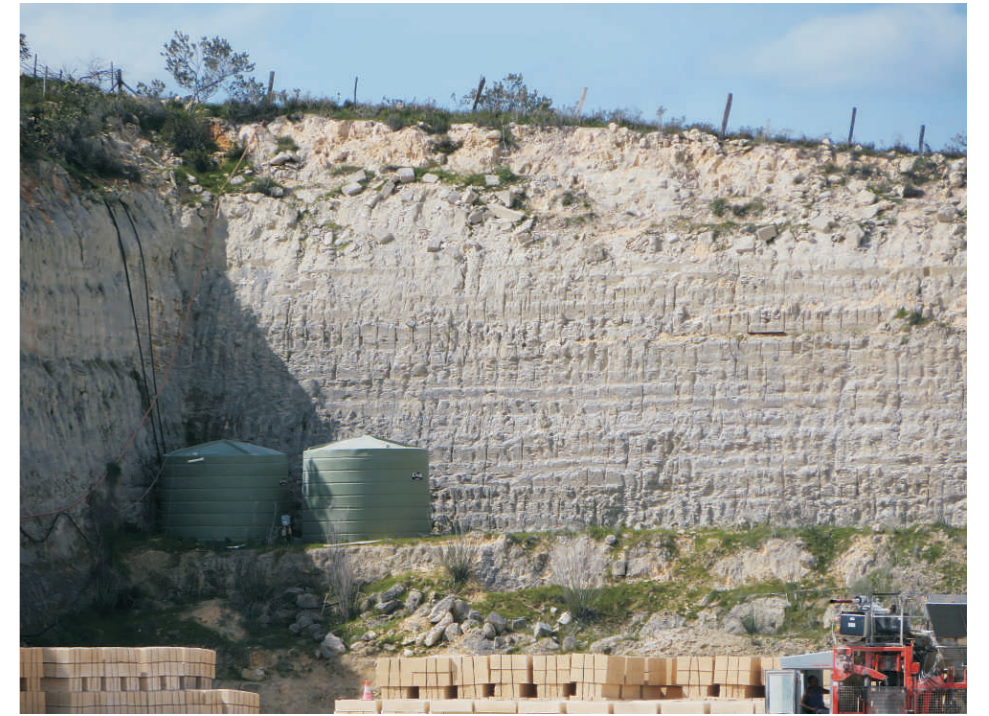
Water tank and eastern face
