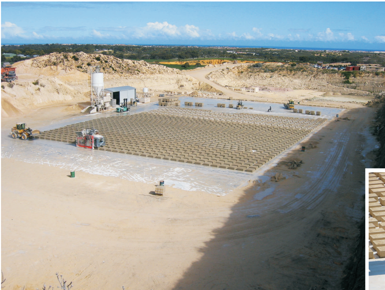
Overview of Lot 6 towards the west across the reconstituted block manufacture floor
