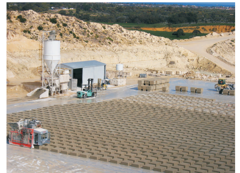
Batch plant and and block making
