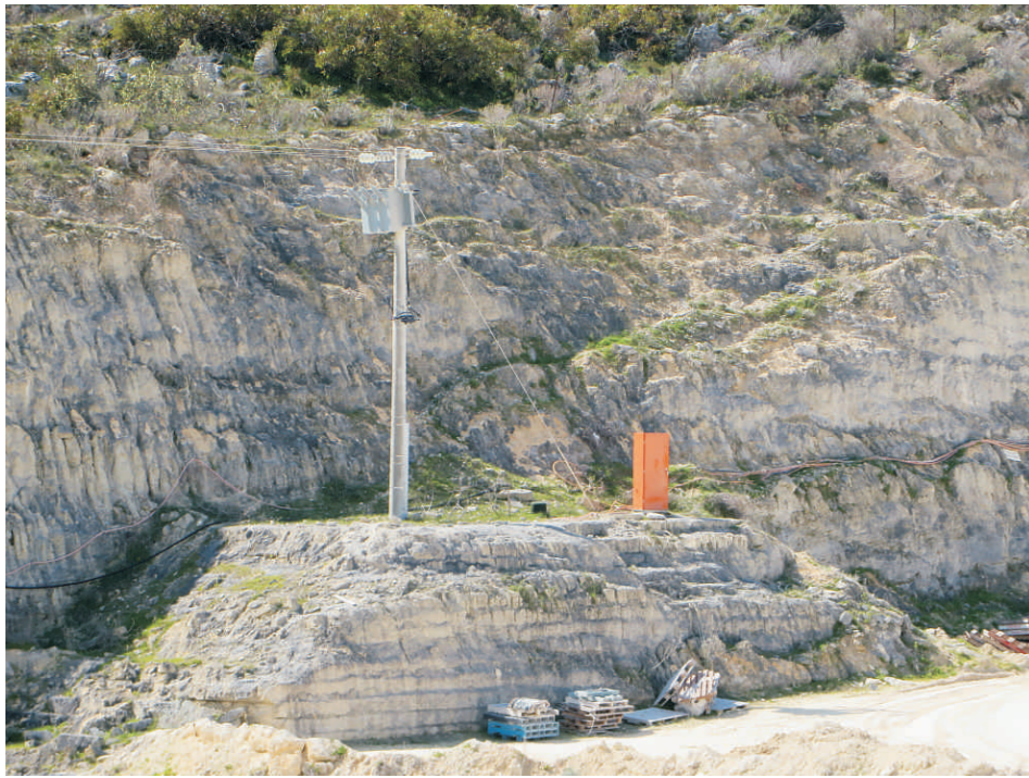
Northern face with electrical facilities
