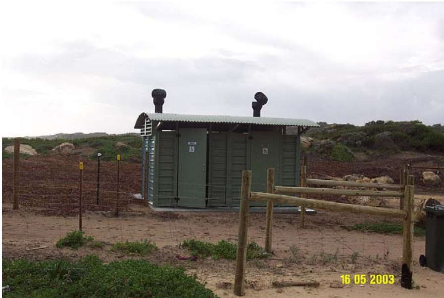
Composting Toilet at Two Rocks
