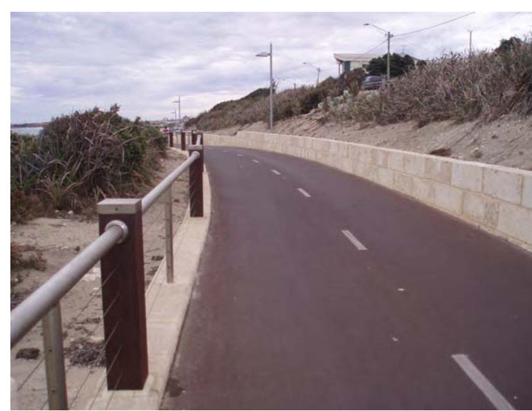
DUAL USE PATH (RED ASPHALT 3m WIDTH)
