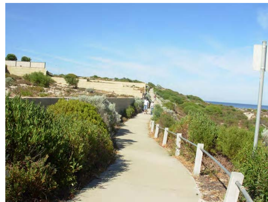
CONCRETE UNIVERSAL ACCESS FOOTPATH
