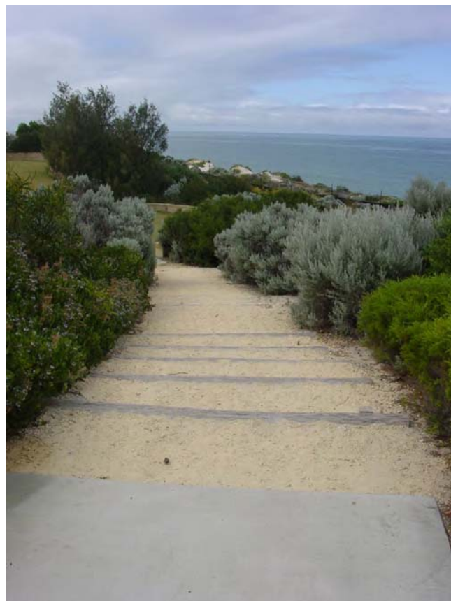
TMBER BEACH ACCESS STEPS
