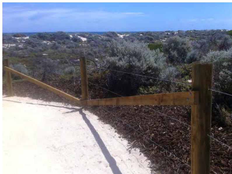
CITY OF WANNEROO APPROVED DUNE & BEACH ACCESS FENCING
