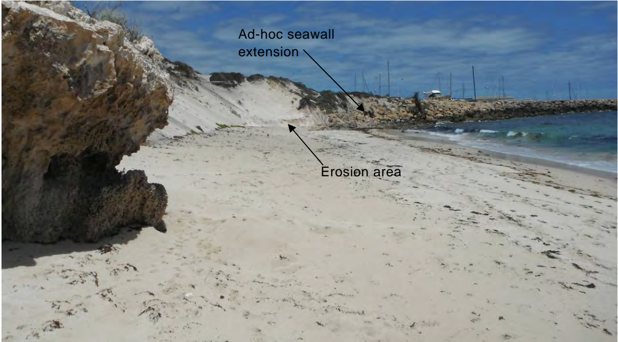
Figure 2.5 - Erosion at the Northern End of the Marina (6/12/12)
