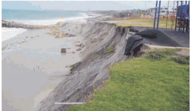
Quinns Rocks foreshore on September 23, when erosion and storm damage prompted the closure of the playground and car park.
