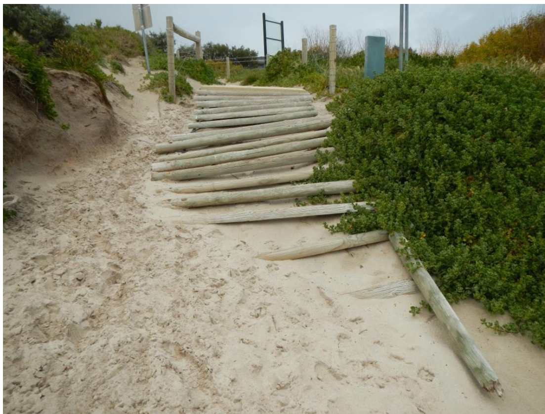
Figure 6-1 Timber log and chain beach access structure (Photo taken 19 September 2016)
