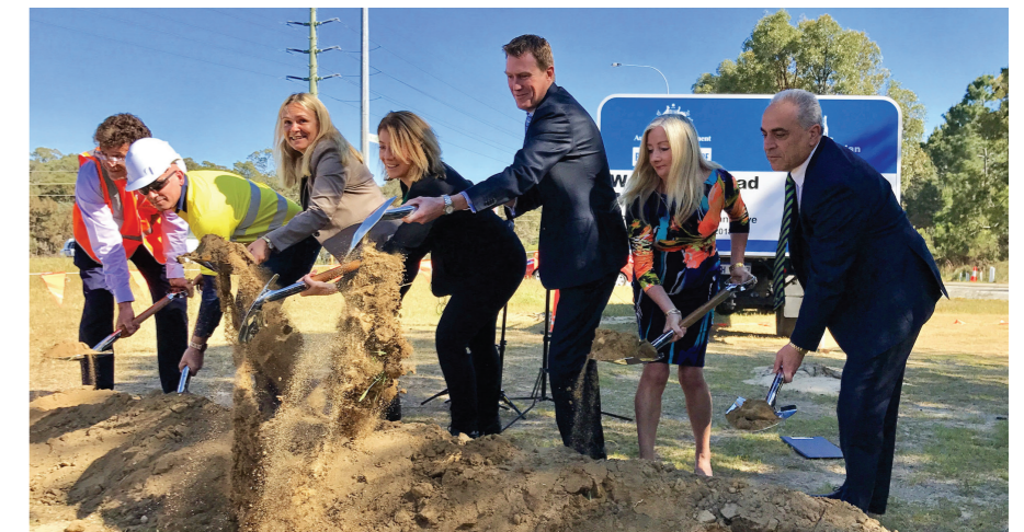
Works for the Wanneroo Road Widening, Joondalup Drive to Flynn Drive, project have commenced with completion scheduled for late 2018.
