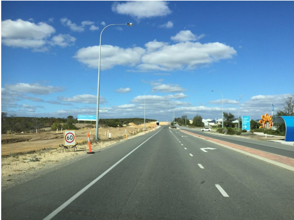
Section 2 – Clearing and Earthworks started / Amberton
