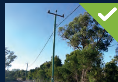
Compliant: cleared buffer zone around power poles
