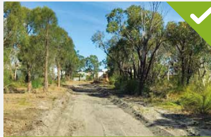
A compliant firebreak needs to be 3m wide and trafficable with a vertical clearance of not less than 4m.
