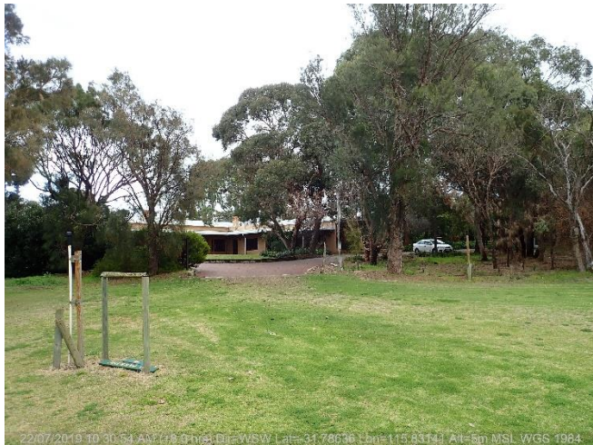
Photo ID: Photo 10 Looking at the reticulated grassland and paved path and building.
