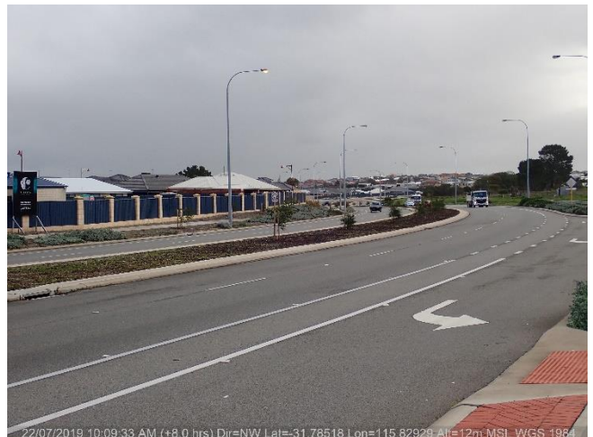
Photo ID: Photo 2 Looking north along Leonore Road at road and houses.
