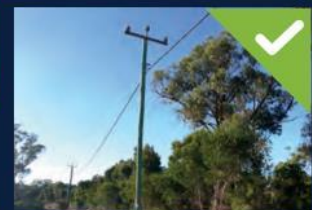
Compliant: cleared buffer zone around power poles
