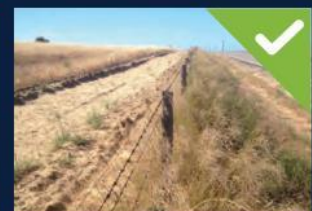
Compliant: mineral earth fire break
