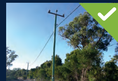
Compliant: cleared buffer zone around power poles
