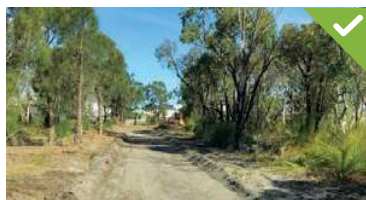
Compliant Fire Break - 3 metre wide trafficable fire break with a vertical clearance of not less than 3.5 metres as close as possible to external boundary.
