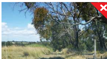
Non-compliant Fire Break - showing grass/weed regrowth and with no vertical 3.5 metre clearance
