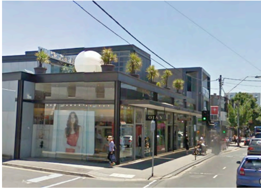
Image 14: Potential for roof terraces on single storey
