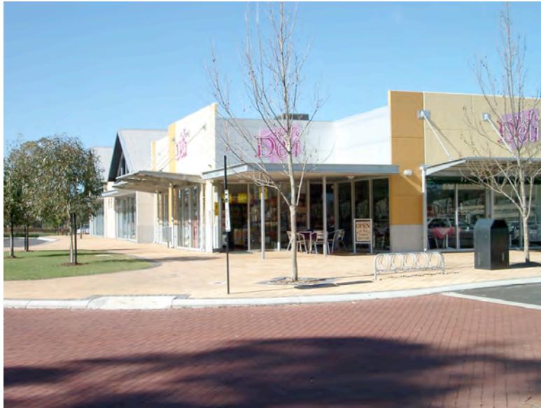
Image 18: 90% weather cover allowing architectural variation
