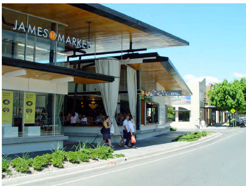
Image 7: Weather protection along street fronts and well defined main entrances improve streetscape and public life.
