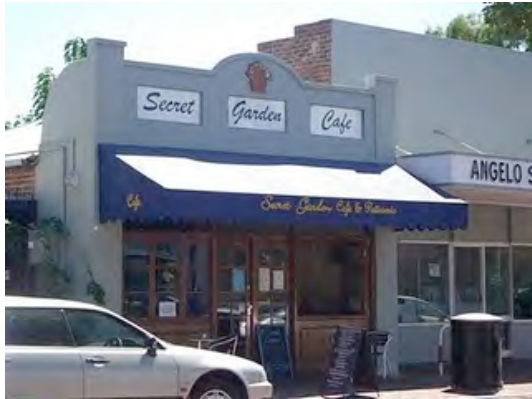
Image 5: Angelo Street, South Perth – Largely single storey development
