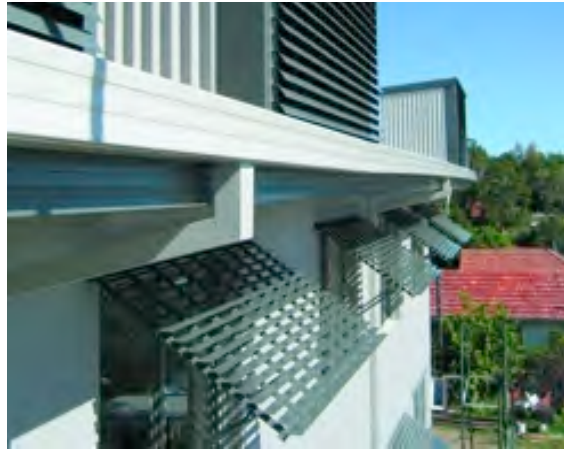
Image 12: Shading in summer and solar access in winter to minimise energy use
