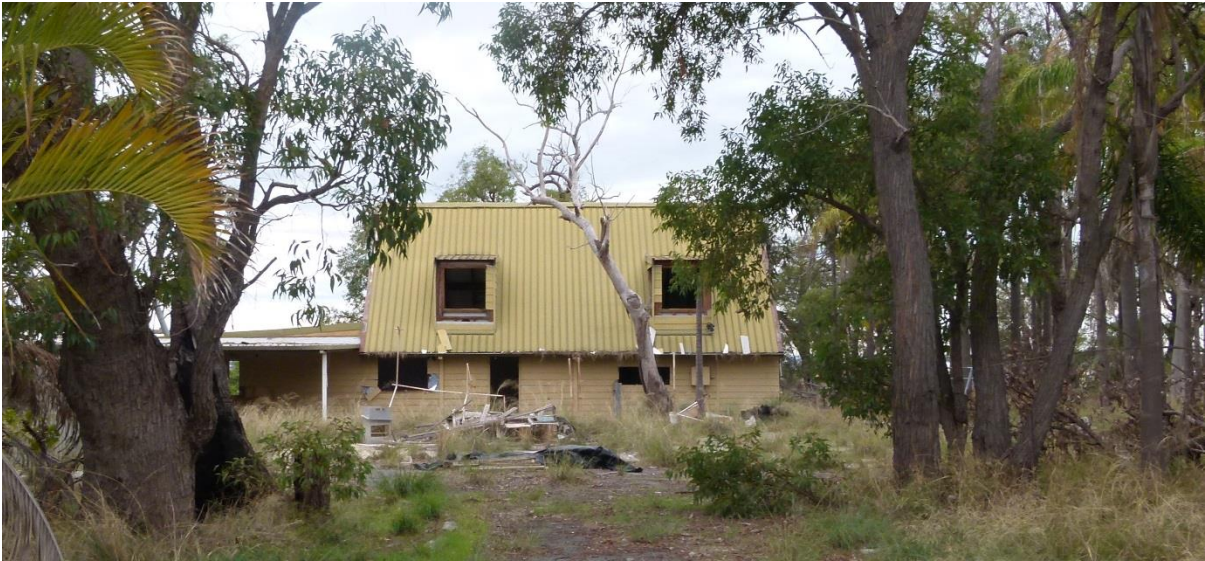
Photograph 3 – Existing double storey building within the subject site to be removed
