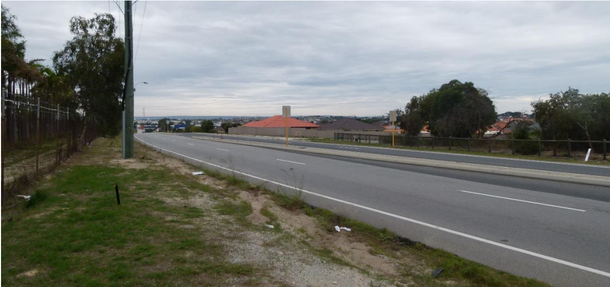
Photograph 6 – View east of Gngara Road along the frontage of the subject site
