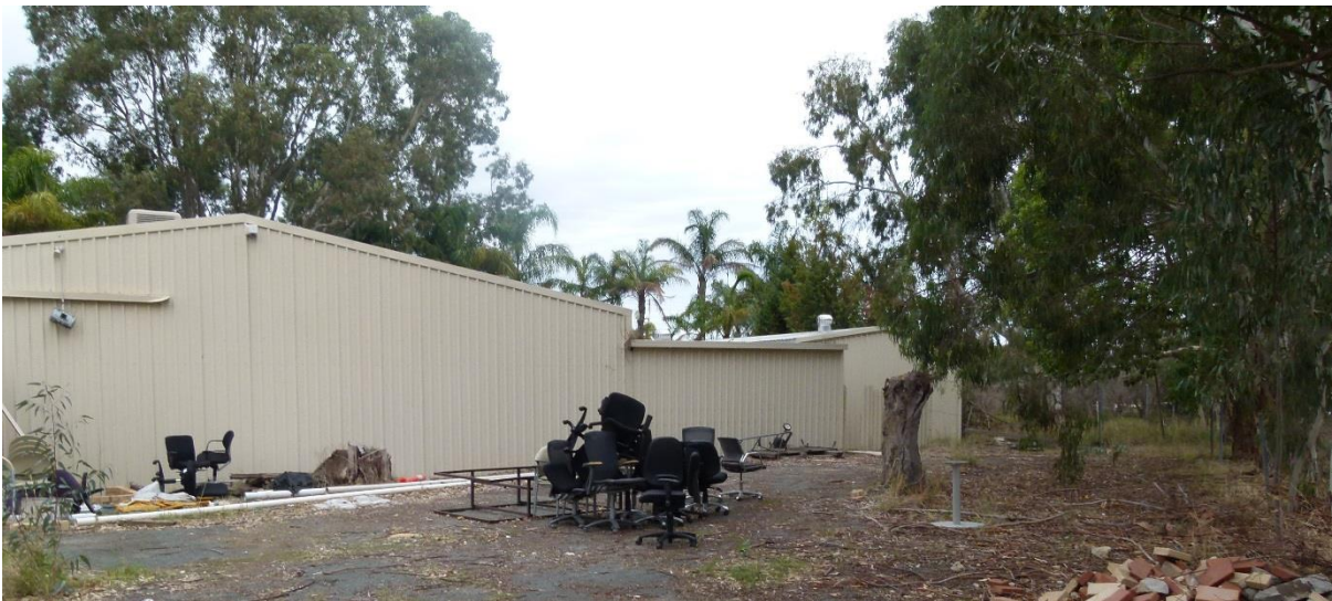
Photograph 4 – Existing shed structures within the subject site to be removed
