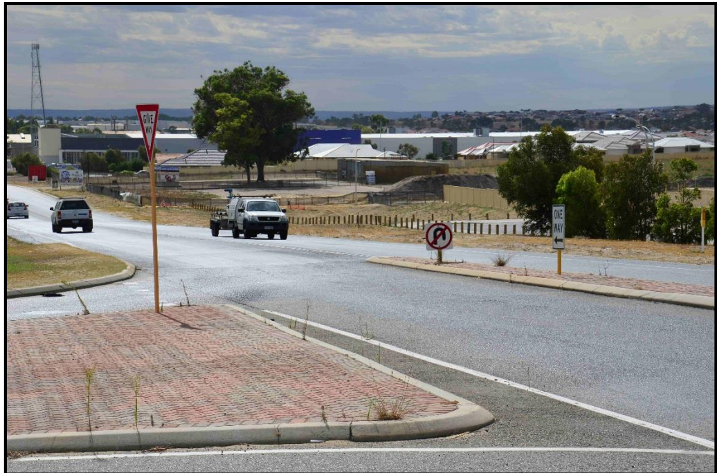
Existing Gngangara Road / Rigali Way intersection
