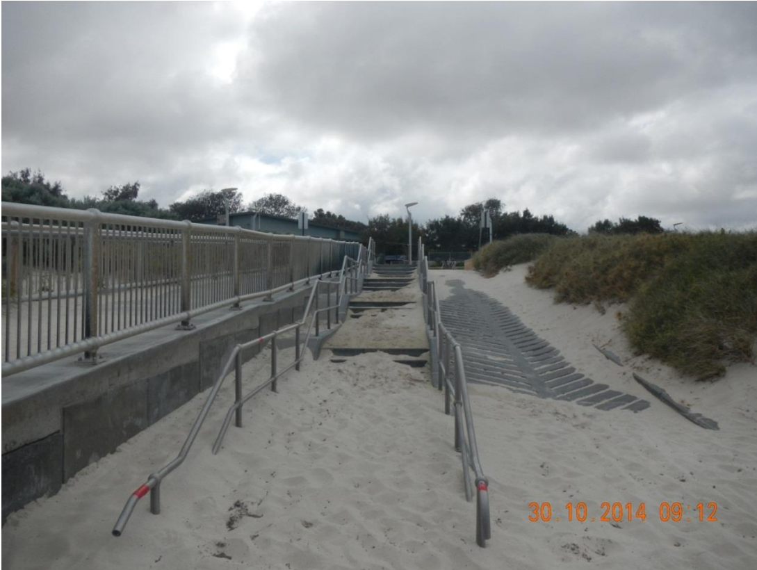
Figure 2-4 Accumulated sand on the beach access from the Surf Life Saving Club
