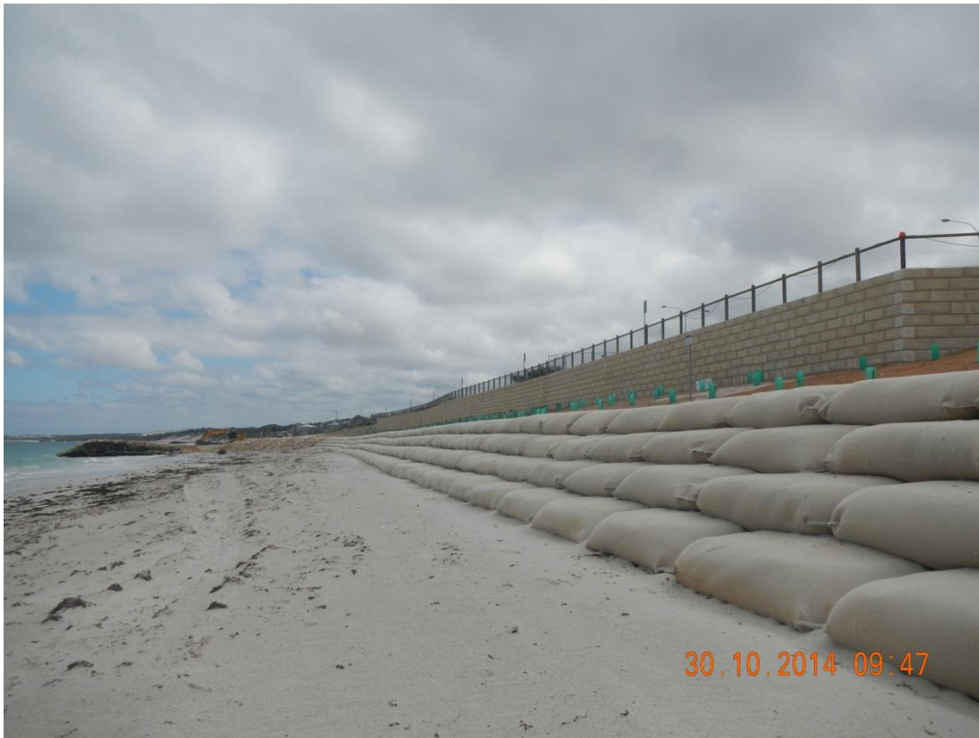
Figure 2-10 The newly constructed GSC revetment and the recently maintained Groyne 1
