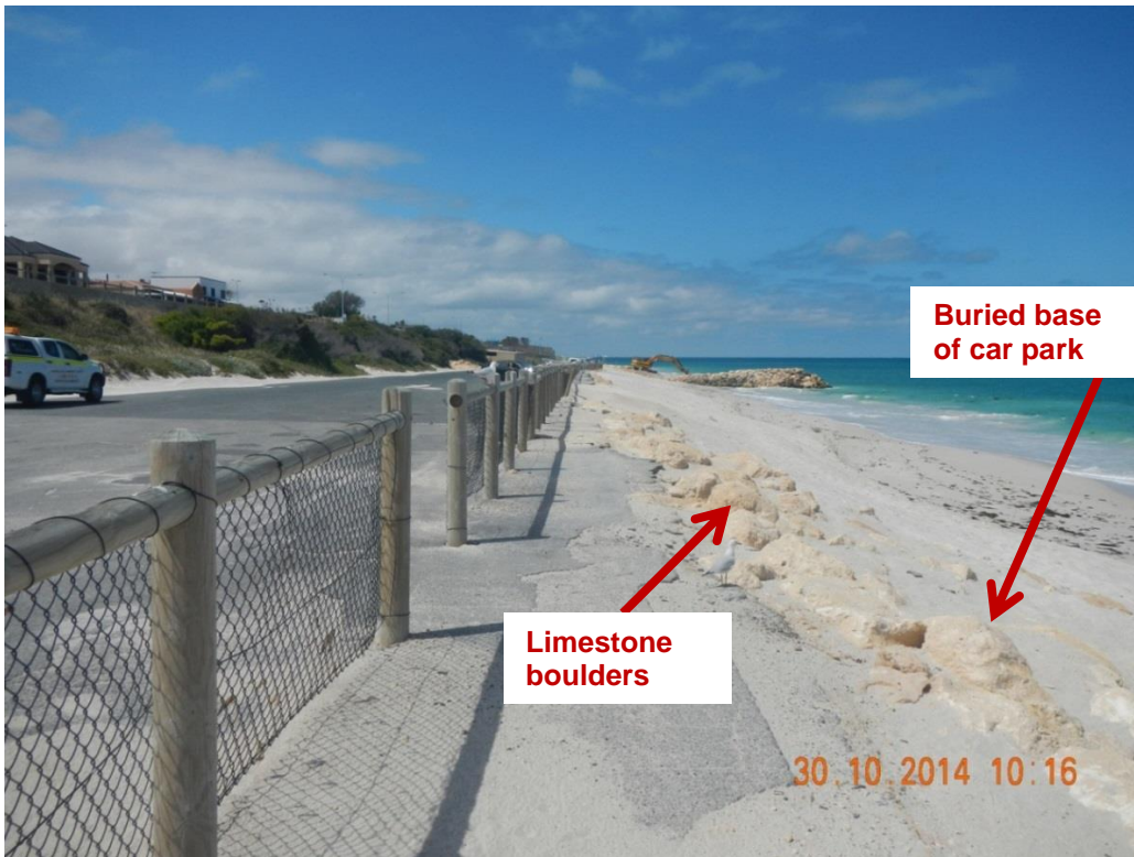
Figure 2-15 Northern end of the car park with the limestone revetment
