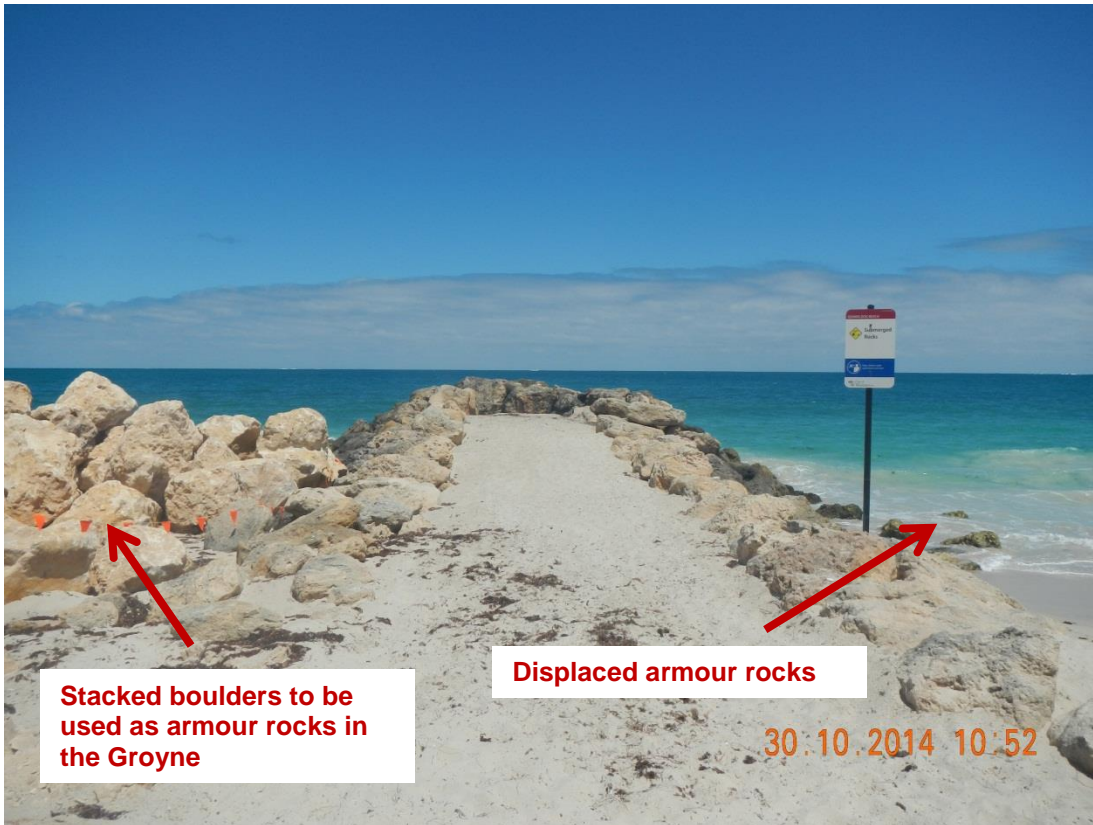
Figure 2-18 Groyne 3 before maintenance works
