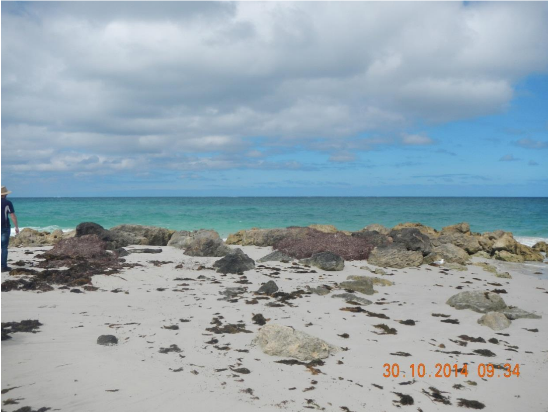
Figure 2-8 The artificial headland, with rocks partially displaced, covered with sand and low crest level
