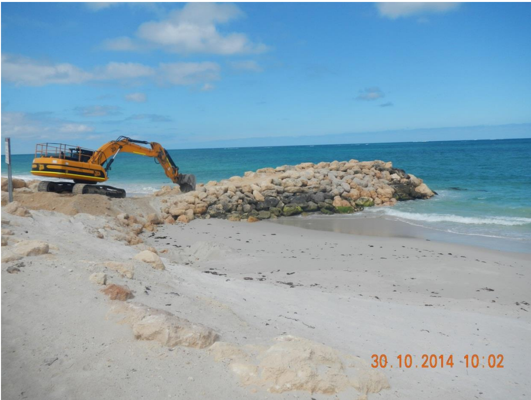
Figure 2-9 Groyne 1 after maintenance
