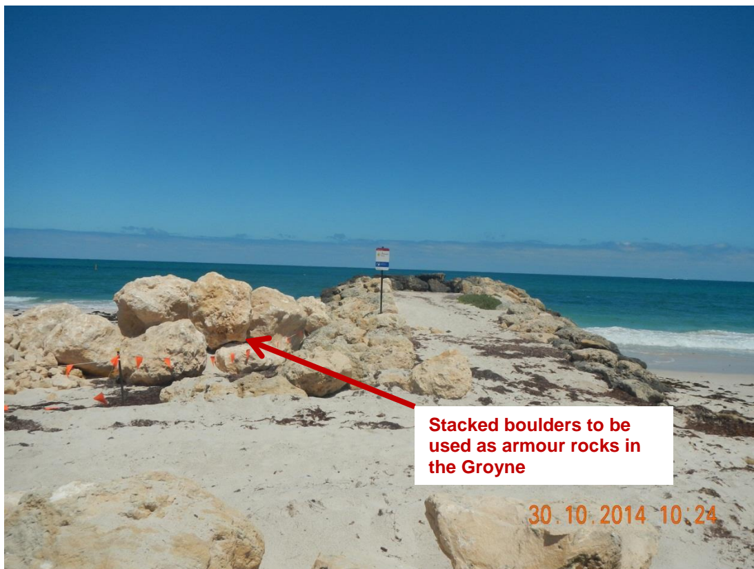
Figure 2-16 Groyne 2 before maintenance works planned for November 2014
