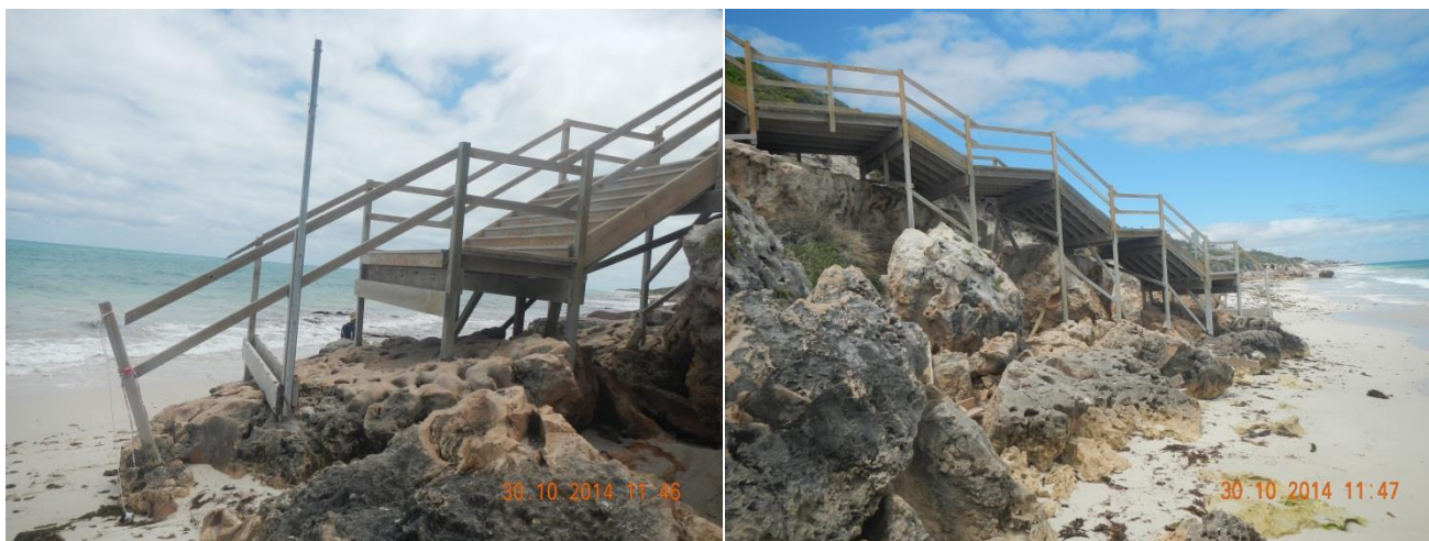
Figure 2-28 Storm damaged stairs
