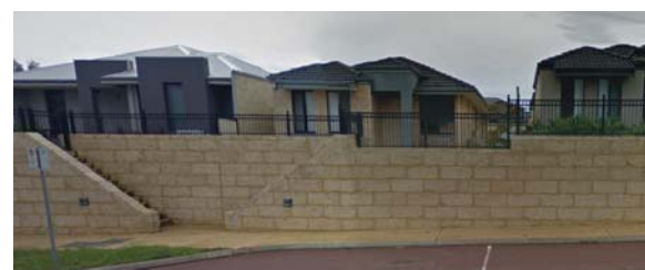
FACE LIMESTONE RETAINING WALLS
