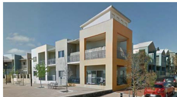
MASONRY FRAMED BALCONIES
