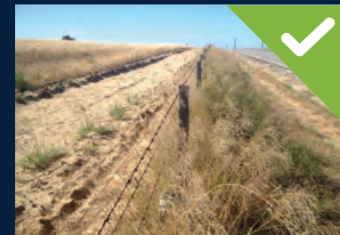
Compliant: mineral earth fire break
