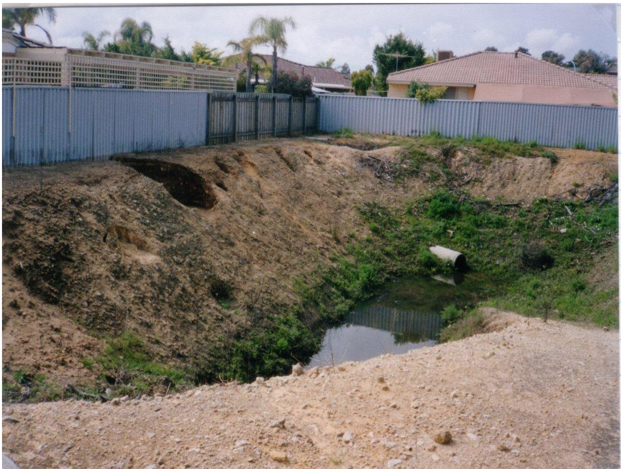
Figure 1 – Road drainage basin at Regatta Drive, Edgewater showing sinkholes on left and at rear.
