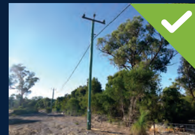
Compliant: cleared buffer zone around power poles
