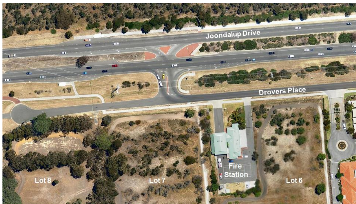
Figure 5: Existing Joondalup Drive intersection
