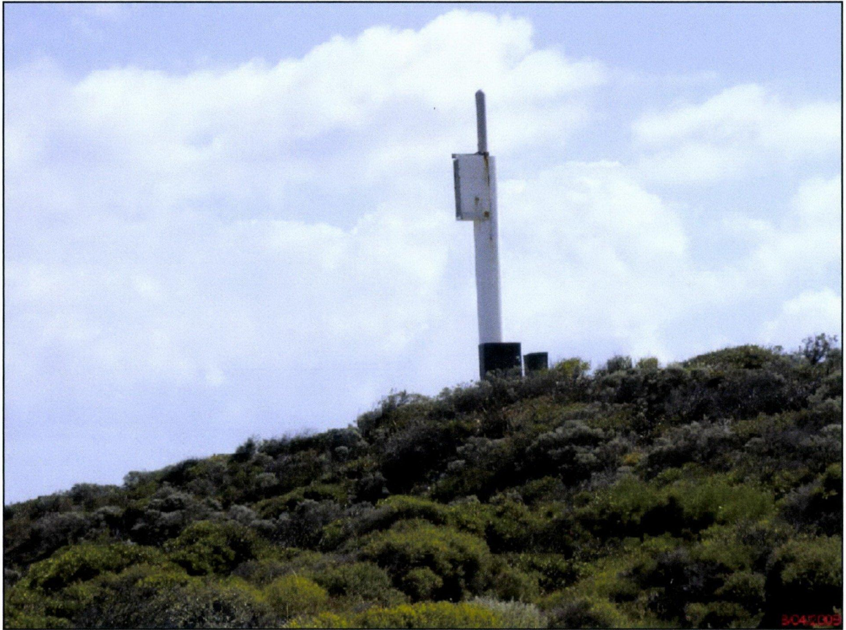
Figure 2 The mobile telecommunications facility at the Department of Transport navigation beacon to be decommissioned
