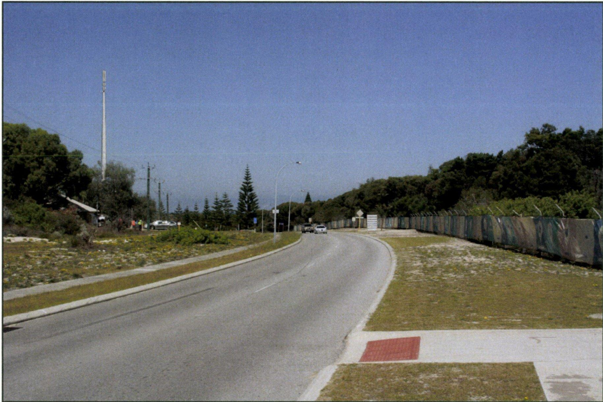
Figure 19 Montage 4 looking south from Lisford Avenue
