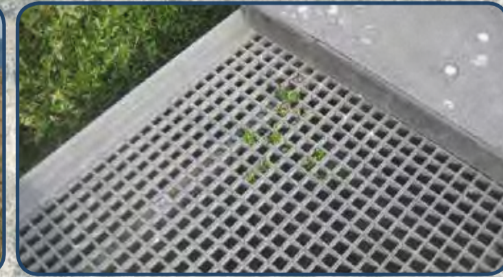
Fibre Reinforced Plastic (FRP): low maintenance materials allow sand to permeate and shrubs to grow through.
