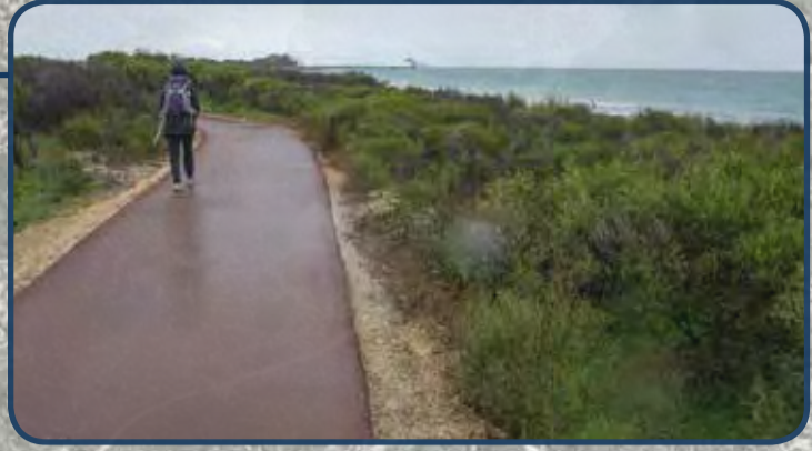
Sealed path: access path network constructed from asphalt on limestone base. Dark colours are recessive in landscapes.
