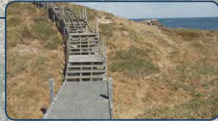
Boardwalk: access boardwalk constructed from composite materials. Recessive colour selections aligned with existing infrastructure.
