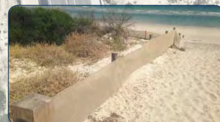
Protection fencing: sand drift dune fencing to restrict access, protect rehabilitation areas and mitigate sand drift.
