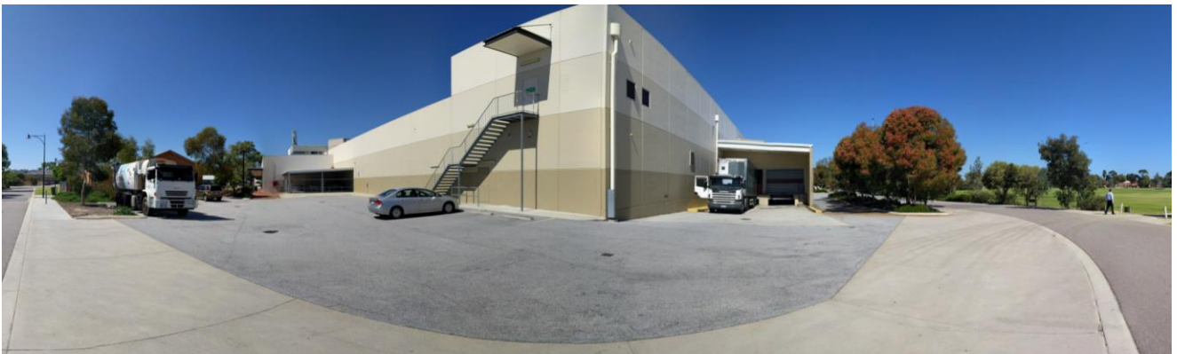
Figure 17 View of the loading dock area (right) and minor car park (left).
