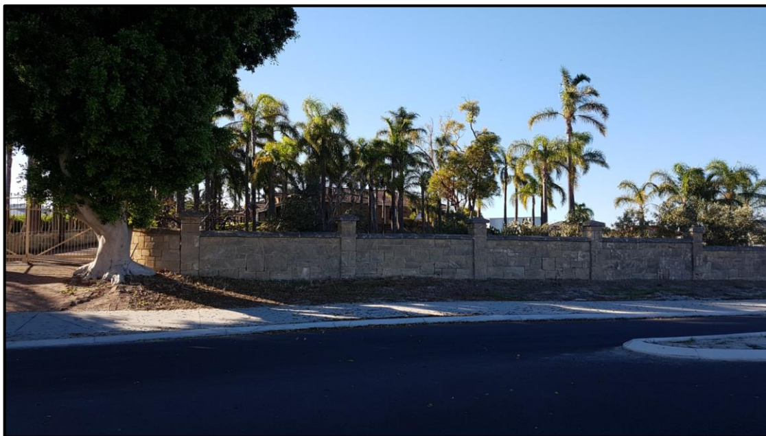
Figure 3: View of Lot 120 looking east from Rangeview Road
