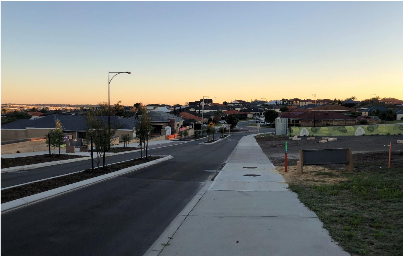
Figure 11 - Rangeview Road current cross section looking north (source: Site visit 25 June 2018)
