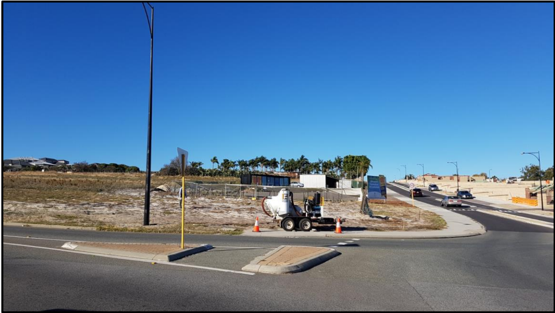
Figure 6: Looking south to the subject site from Kingsway
