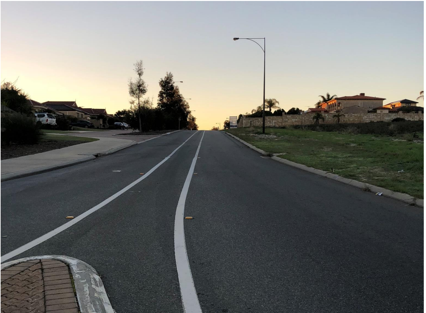
Figure 8 - Kingsway current cross section looking east (source: Site visit 25 June 2018)
