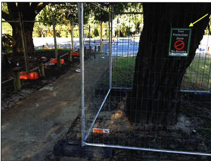
Figure 3. Protective fencing comprised of 1.8m high chain-wire mesh panels and signage providing information (see arrow) regarding access within the fencing should be erected prior to the commencement of construction activities that involve machinery and have the potential for collision injury.
