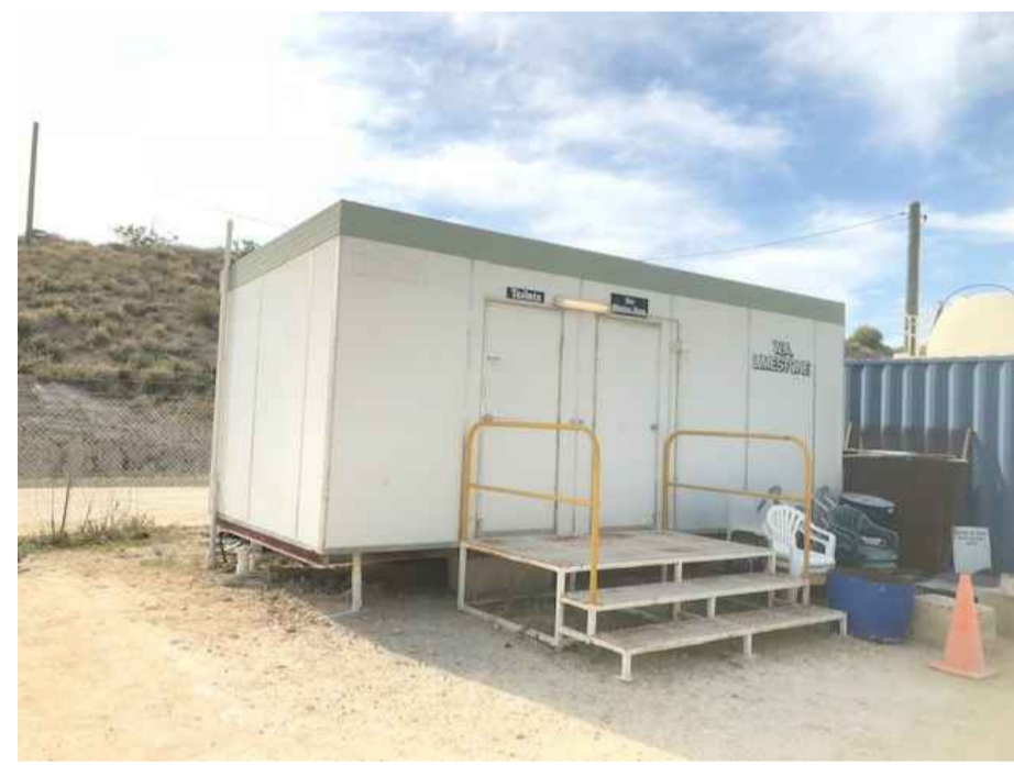
PHOTO - TOILETS/SITE OFFICE
