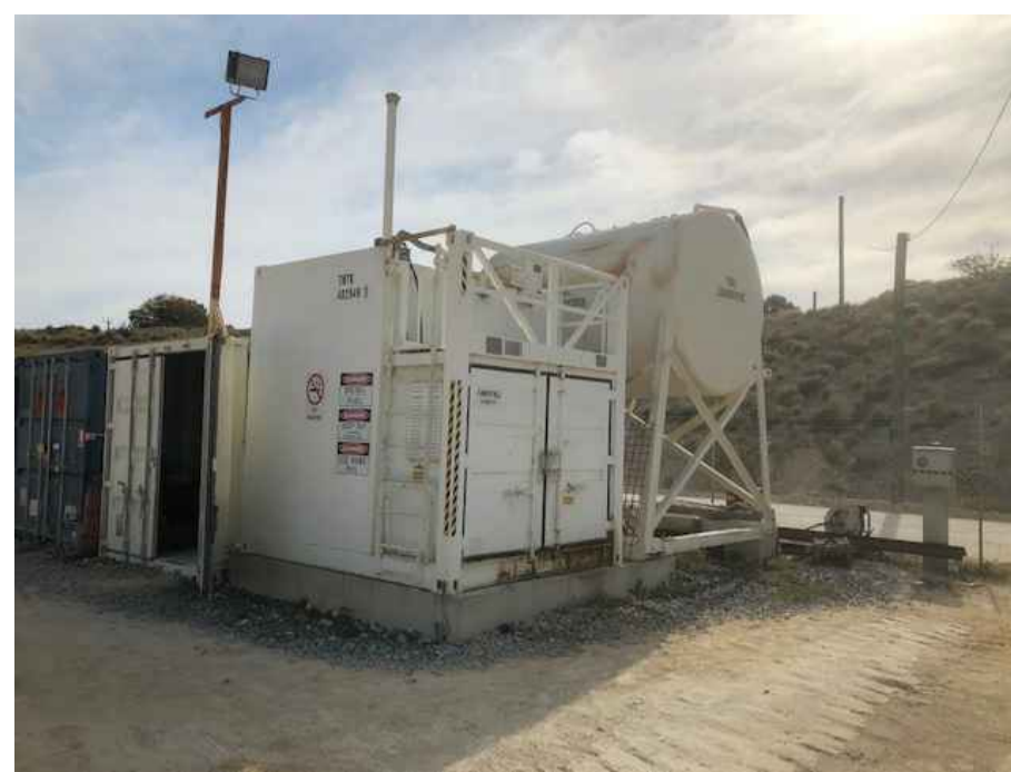
PHOTO - FUEL/MAINTENANCE SUPPLIES
