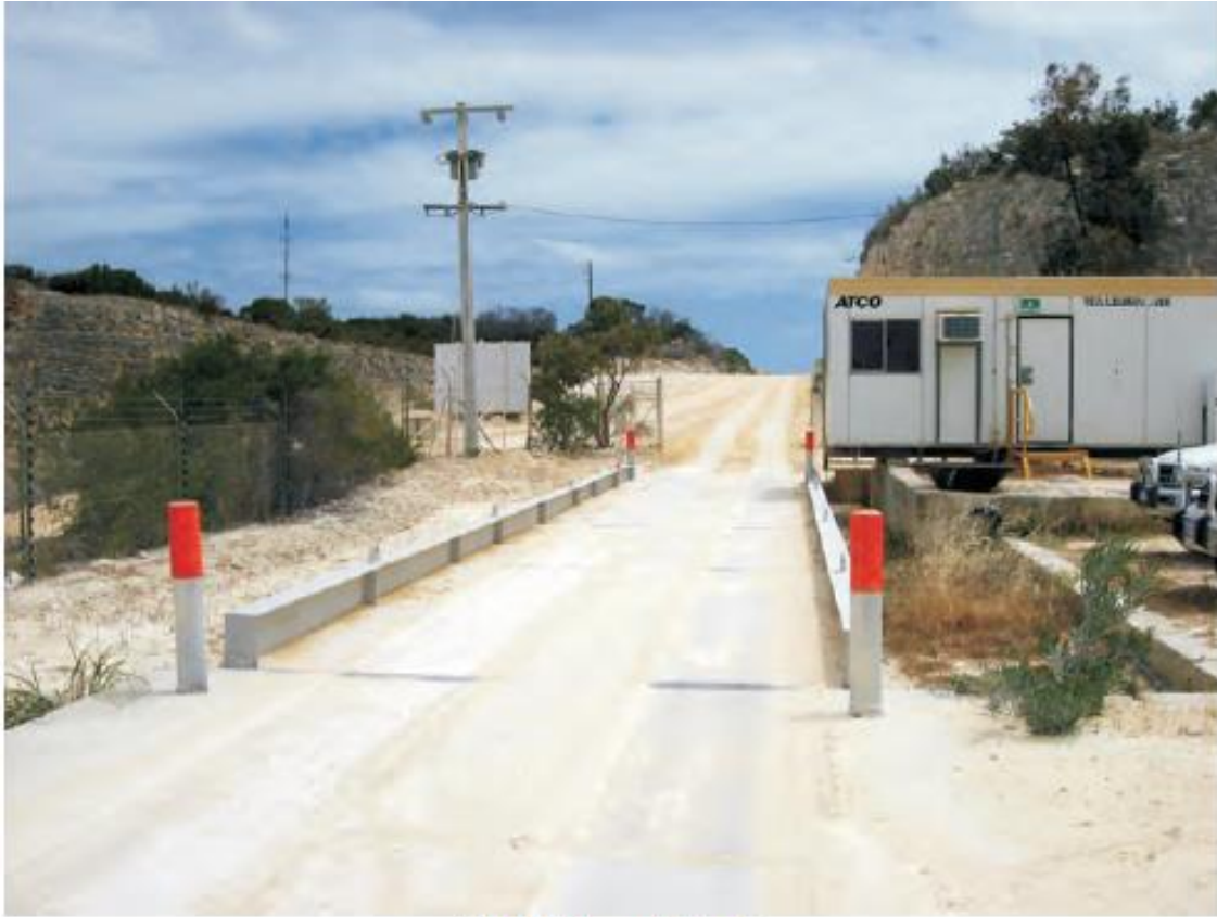
Weighbridge and site office
