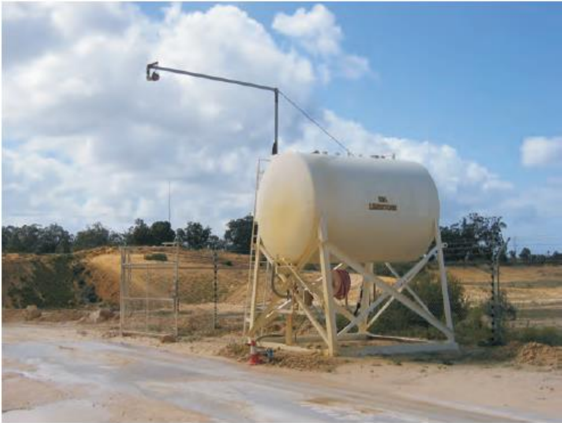
Truck wet down facility near the weighbridge
