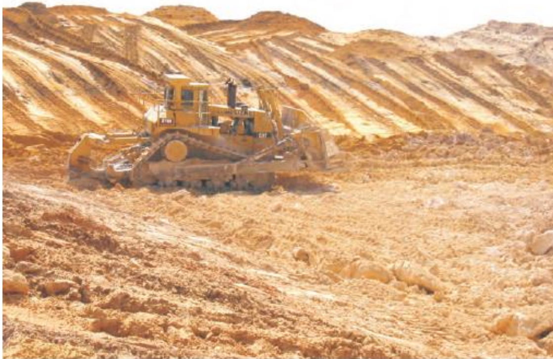
Bulldozer ripping limestone for excavation
