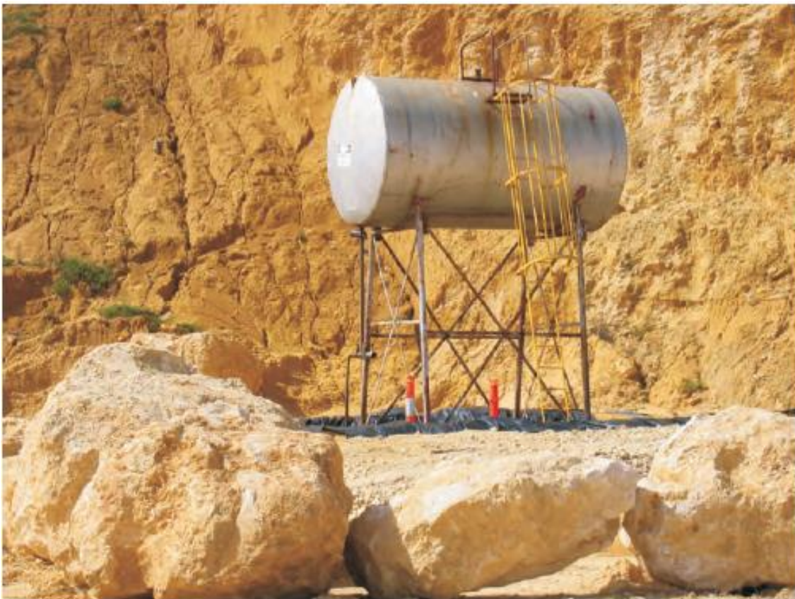
Fuel tank located in a bunded and lined facility
