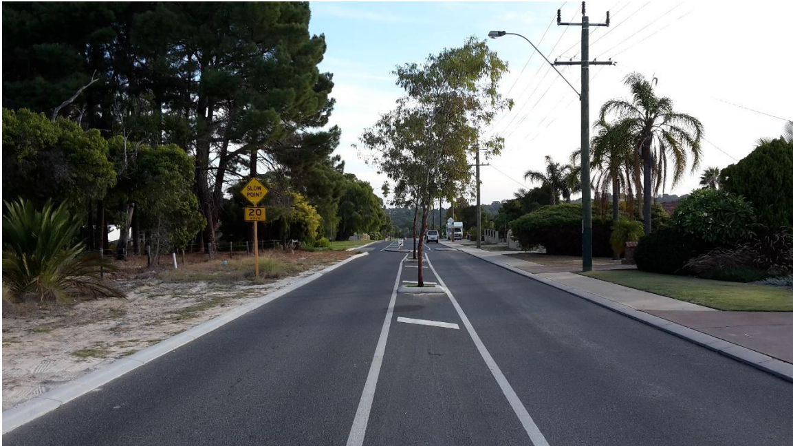
Figure 3. Westbound view along San Rosa Road in the vicinity of subject site
