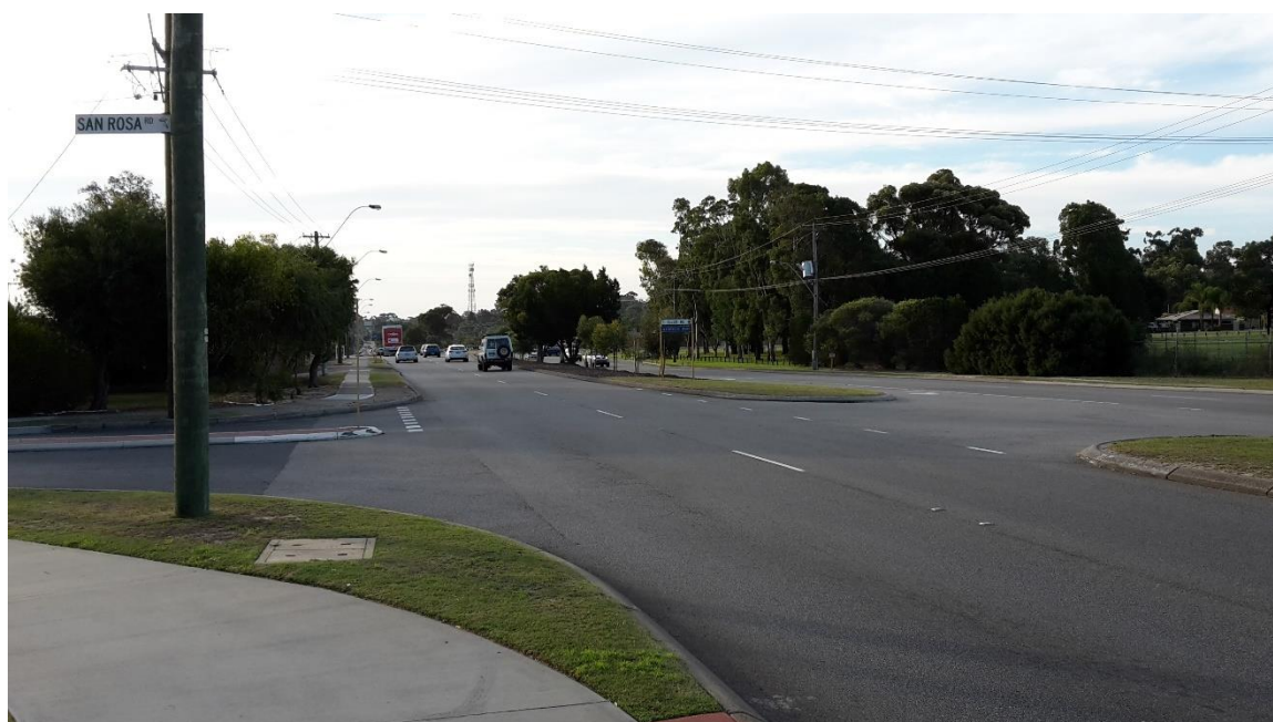
Figure 8. Northbound view along Wanneroo Road from San Rosa Road intersection
