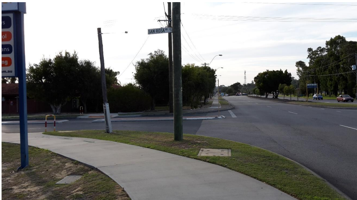
Figure 6. Northbound view along Wanneroo Road from San Rosa Road intersection
