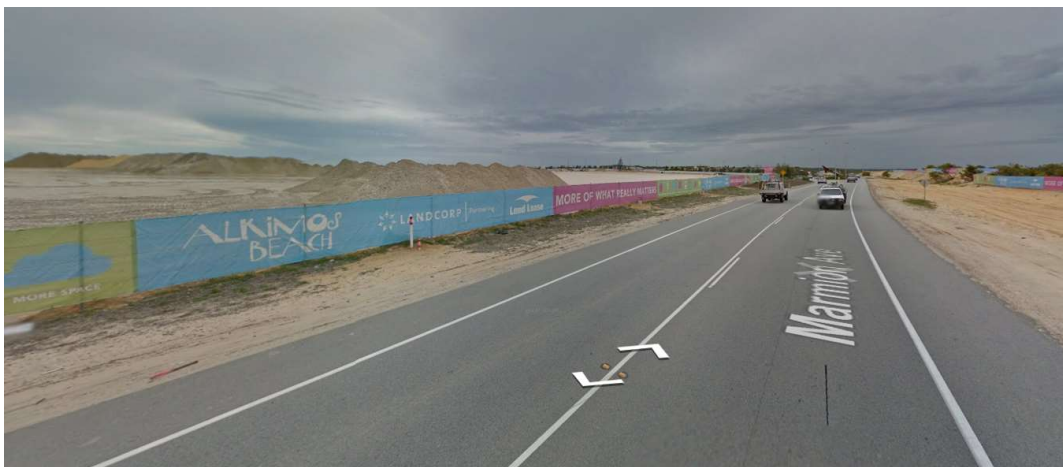
Figure 2: Marmion Avenue adjacent to the subject site (looking north)
