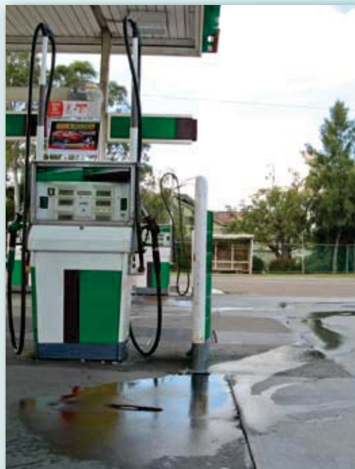
Picture shows a defective forecourt design with oils and fuels discharging directly to the street drain.
