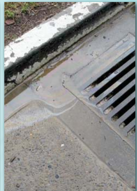
Unseemly & highly visible hydrocarbons polluting the stormwater. The concentration in the picture is in excess of 100ppm
