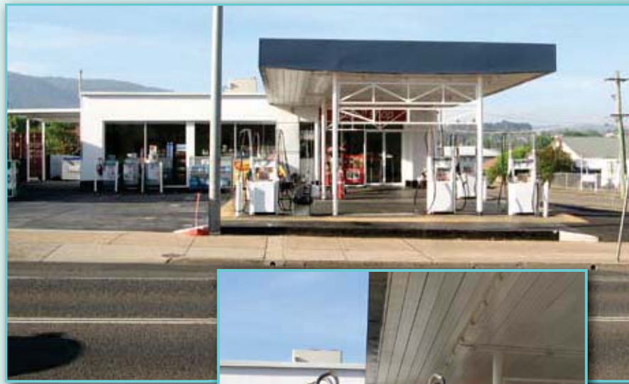
Picture shows an under-sized canopy with fuel pumps outside the canopy dripline
