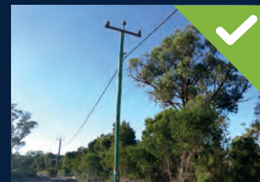
Compliant: cleared buffer zone around power poles
