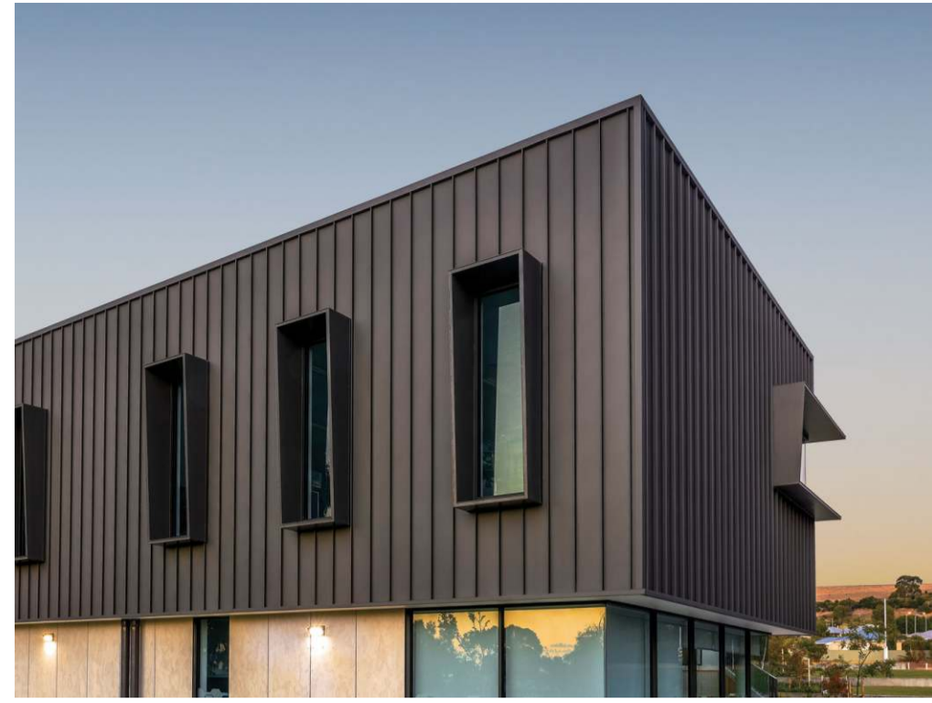
Dark/charcoal metal profile cladding to external facades. Maxline 340.
