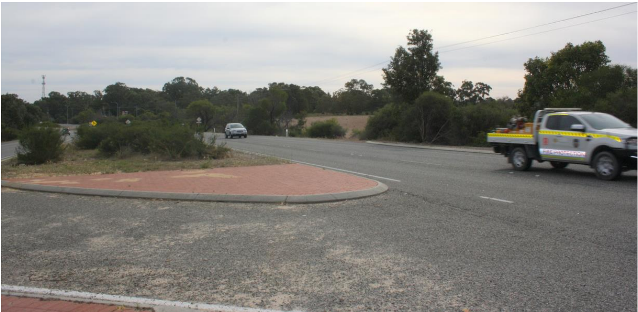
Photograph 8 – Sight line from right and U turn facility at Train Rd to southbound Wanneroo Rd traffic restricted by vegetation in median island
