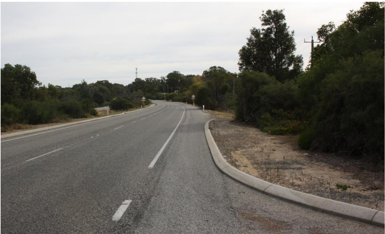
Photograph 9 – Example of sealed shoulders on both sides of Wanneroo Road that are designated as formal cycle routes
