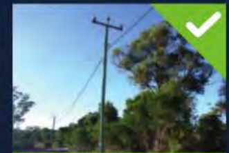
Compliant: cleared buffer zone around power poles
