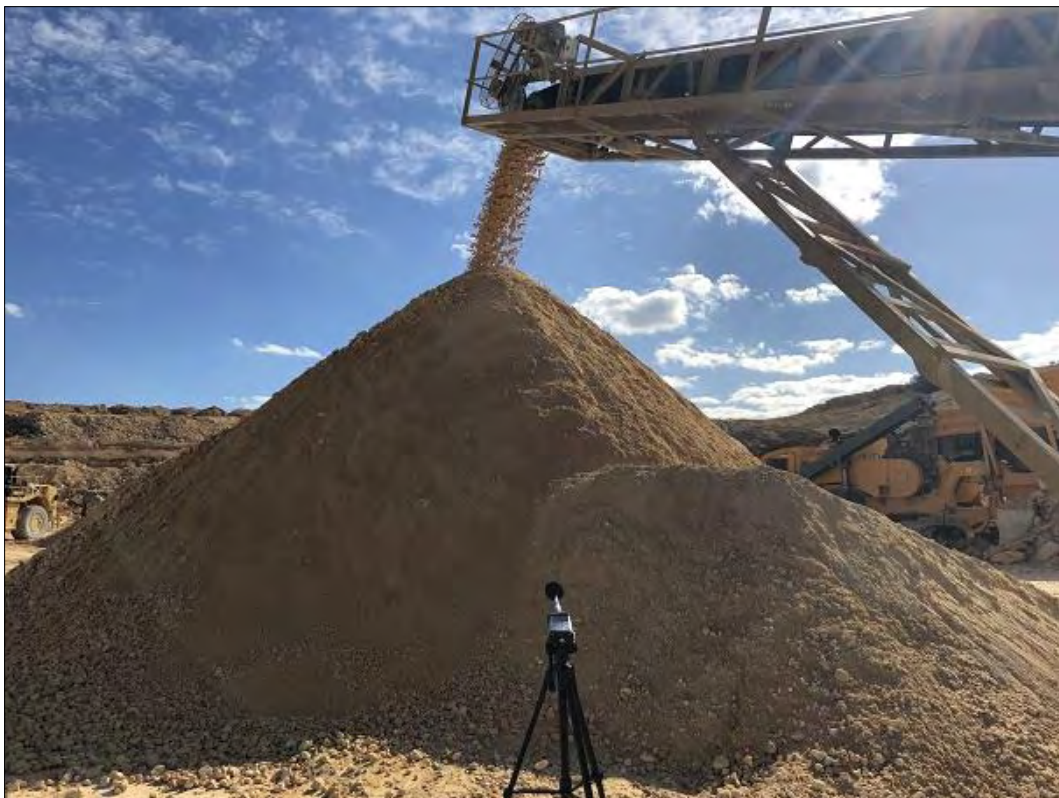
Photo 10: Stockpile – Existing quarry at Lot 501 Wattle Avenue, Nowergup
