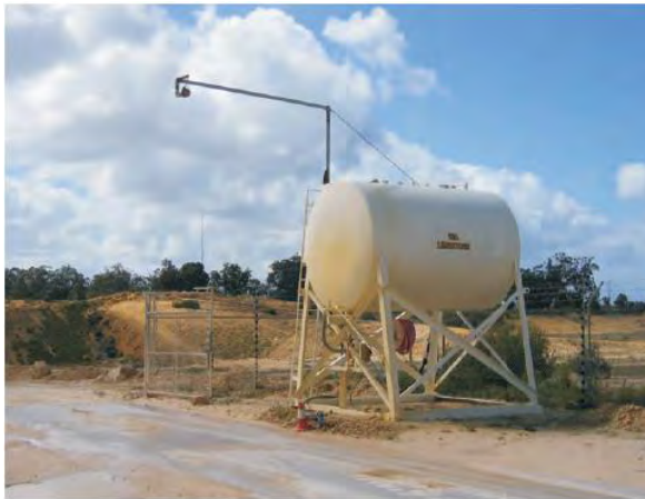
Truck wet down facility near the weighbridge
