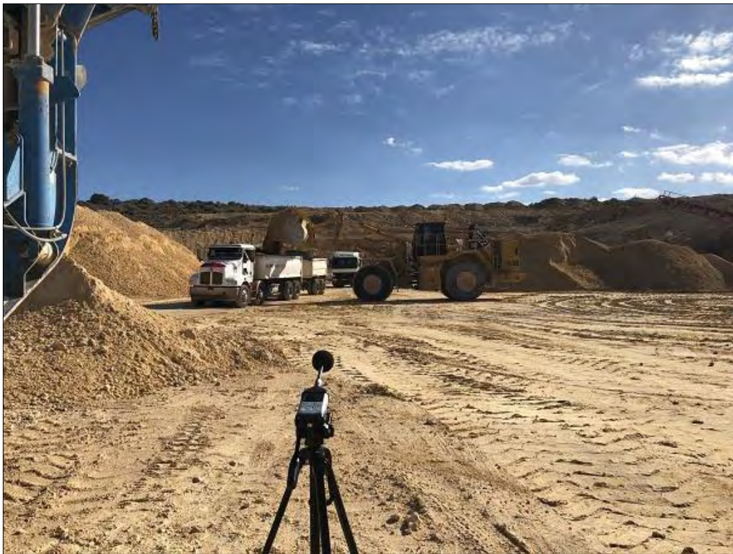
Photo 11: Loader and product truck – Existing quarry at Lot 501 Wattle Avenue, Nowergup
