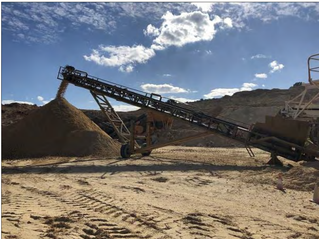
Photo 6: Conveyor – Existing quarry at Lot 501 Wattle Avenue, Nowergup
