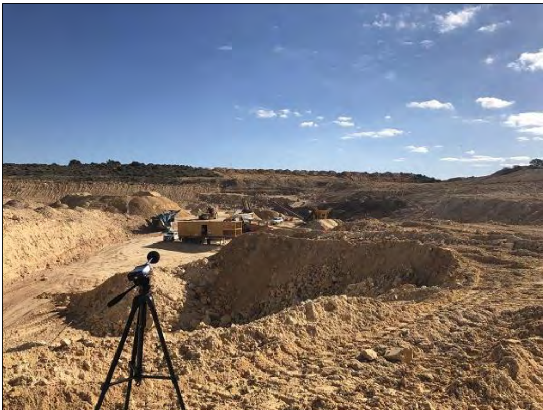
Photo 12: View from top of existing quarry at Lot 501 Wattle Avenue, Nowergup
