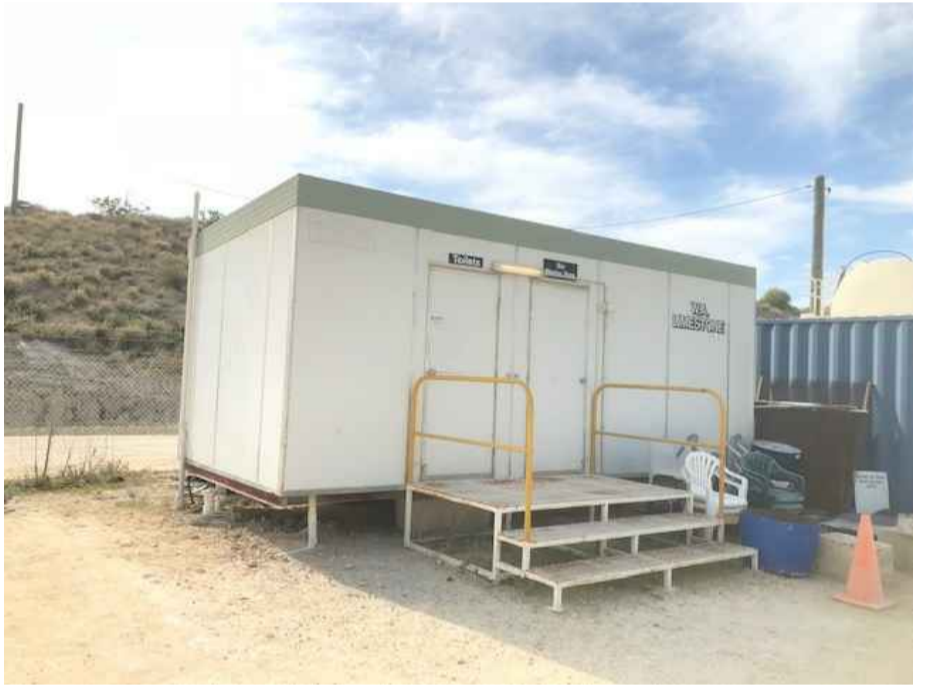
PHOTO - TOILETS/SITE OFFICE
