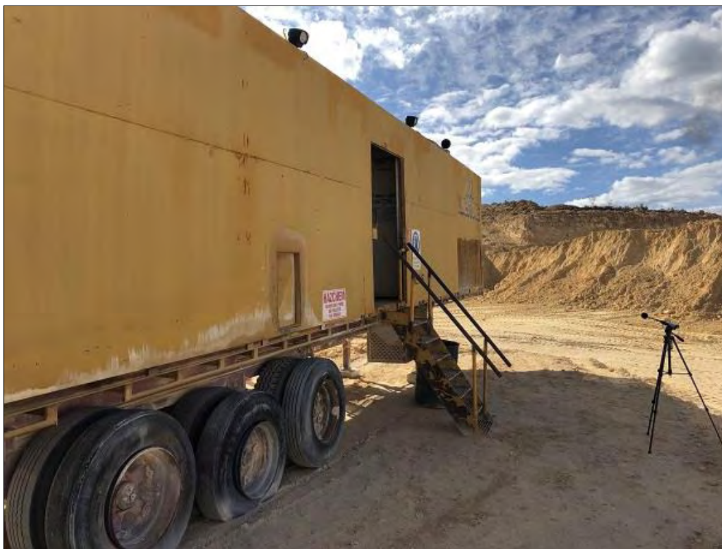
Photo 7: Generator – Existing quarry at Lot 501 Wattle Avenue, Nowergup
