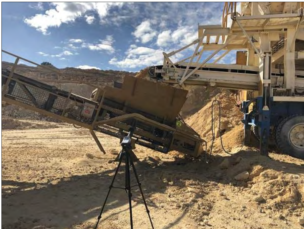
Photo 8: Conveyor – Existing quarry at Lot 501 Wattle Avenue, Nowergup
