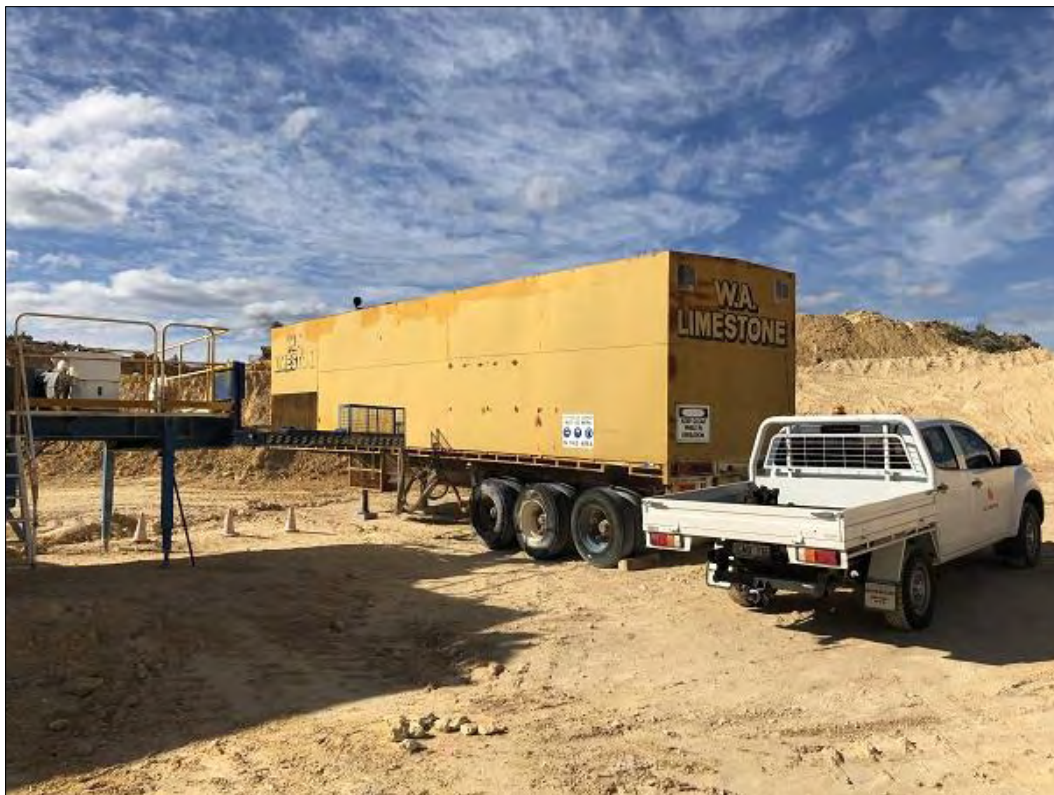
Photo 4: Generator – Existing quarry at Lot 501 Wattle Avenue, Nowergup
