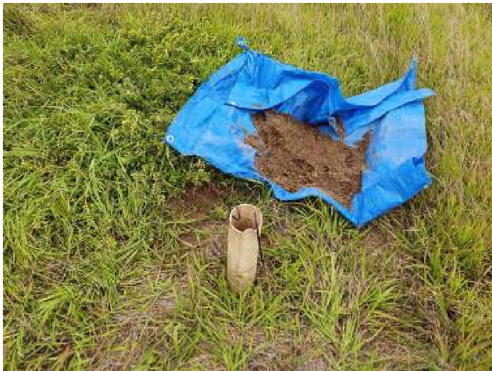
Photograph 7: IT02 (Unit 1a SAND FILL) – Inverse auger hole test setup
