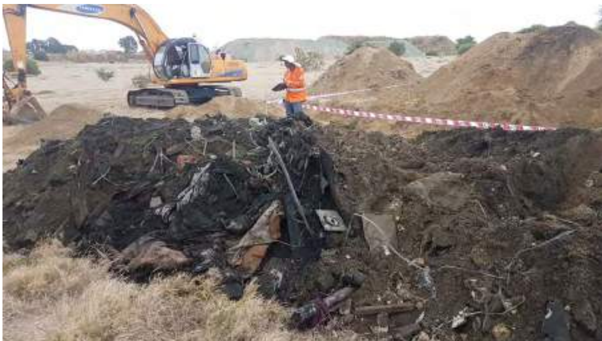
Photograph 1: Test Pitting
