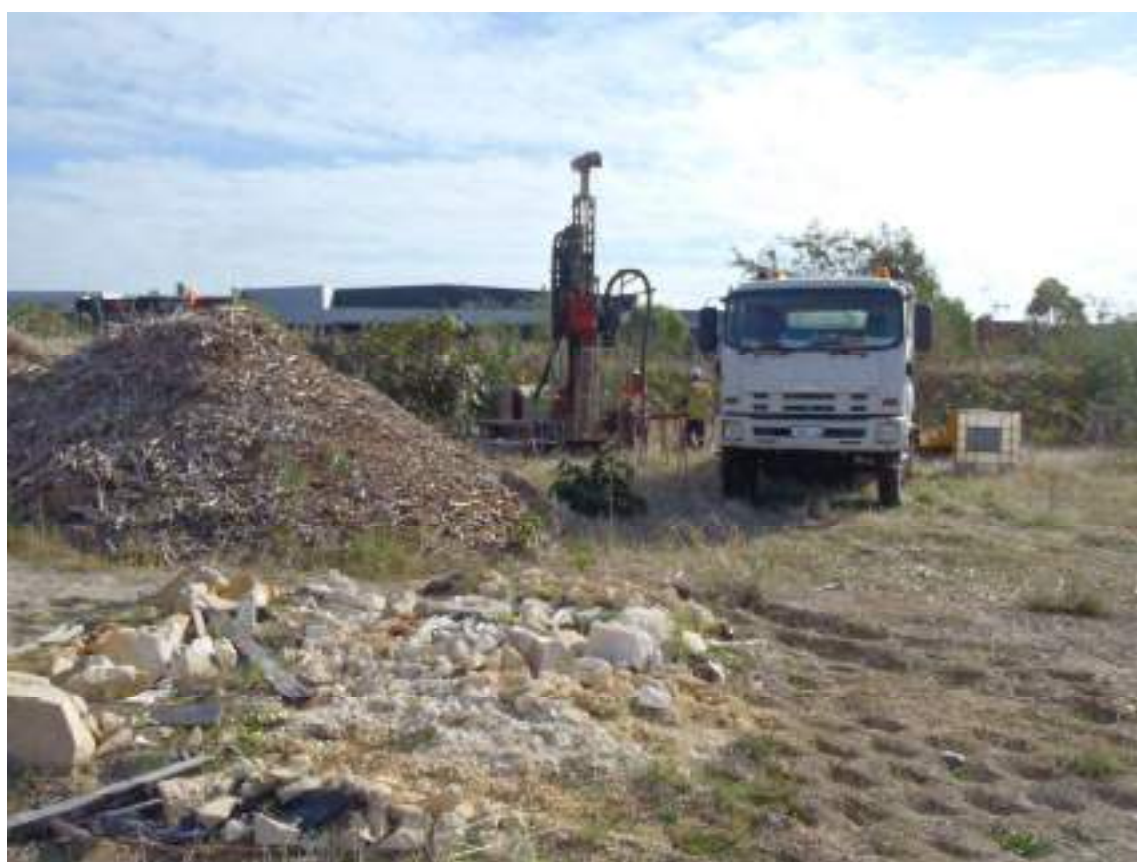
Photograph 4: Borehole Drilling
