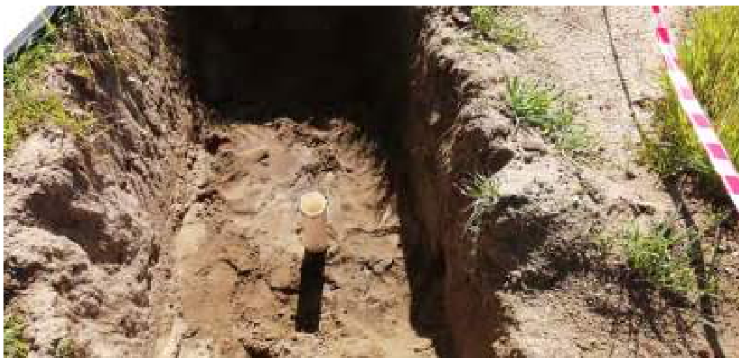
Photograph 9: Inverse auger hole setup for testing in Unit 1C (Screened FILL) present below surficial layer of Unit 1A (SAND FILL)
