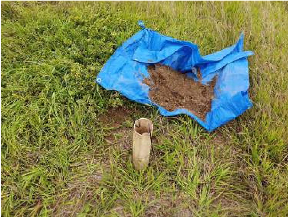
Photograph 1: IT02 (Unit 1a SAND FILL) – Inverse auger hole test setup
