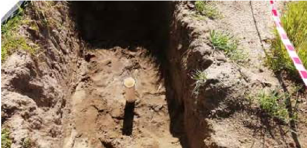
Photograph 3: Inverse auger hole setup for testing in Unit 1C (Screened FILL) present below surficial layer of Unit 1A (SAND FILL)
