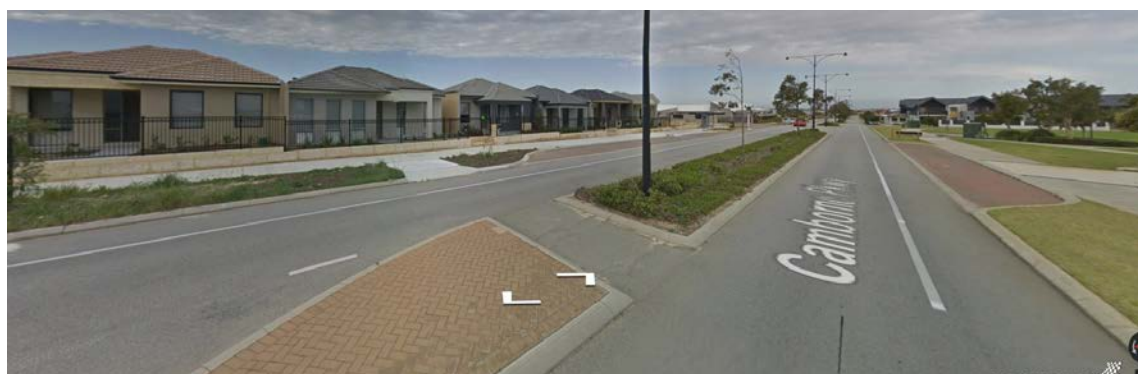
Figure 3: Camborne Parkway in the vicinity of the subject site – Looking South
