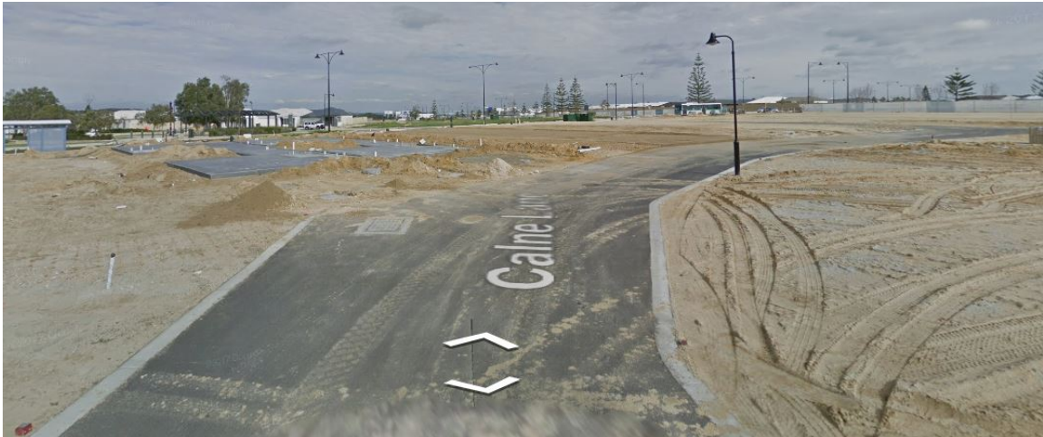
Figure 4: Calne Lane in the vicinity of the subject site – Looking East
