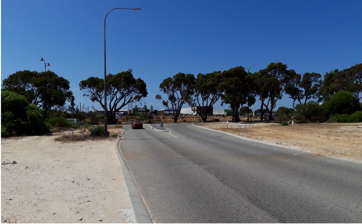
Figure 5: Northbound view along Kakadu Road in the vicinity of future site's crossover
