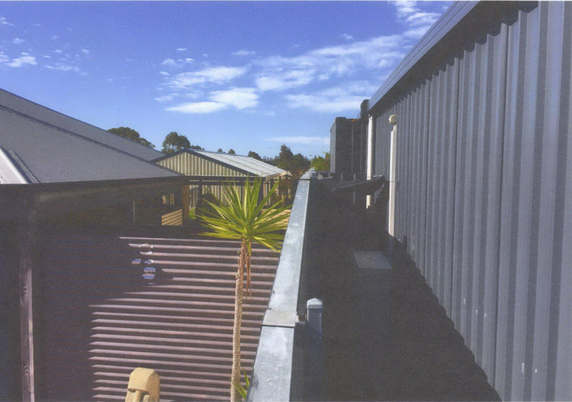
SIDE OF HOUSE VIEW
