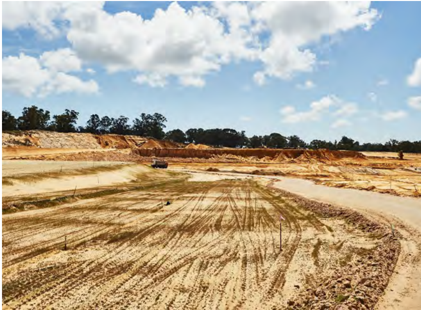
Typical excavation with a completed floor
