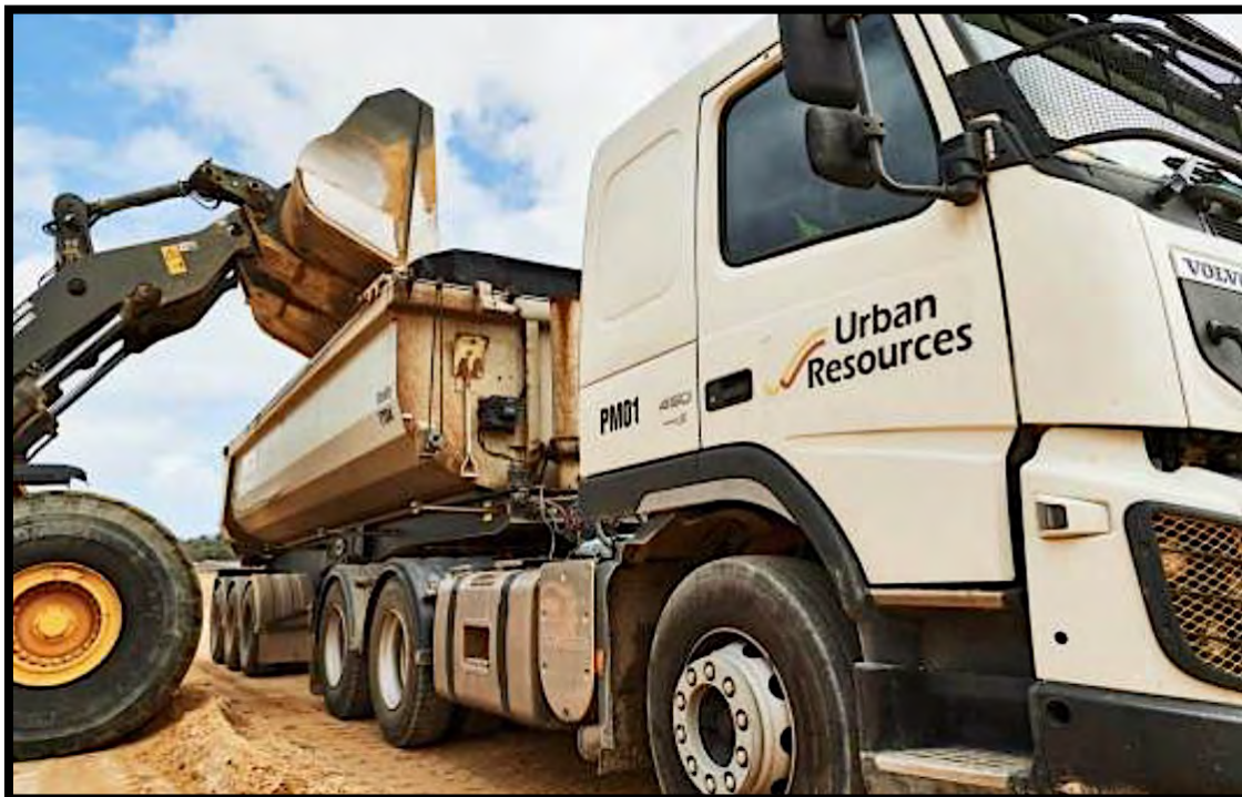
Figure 8: Loading sand onto road truck
