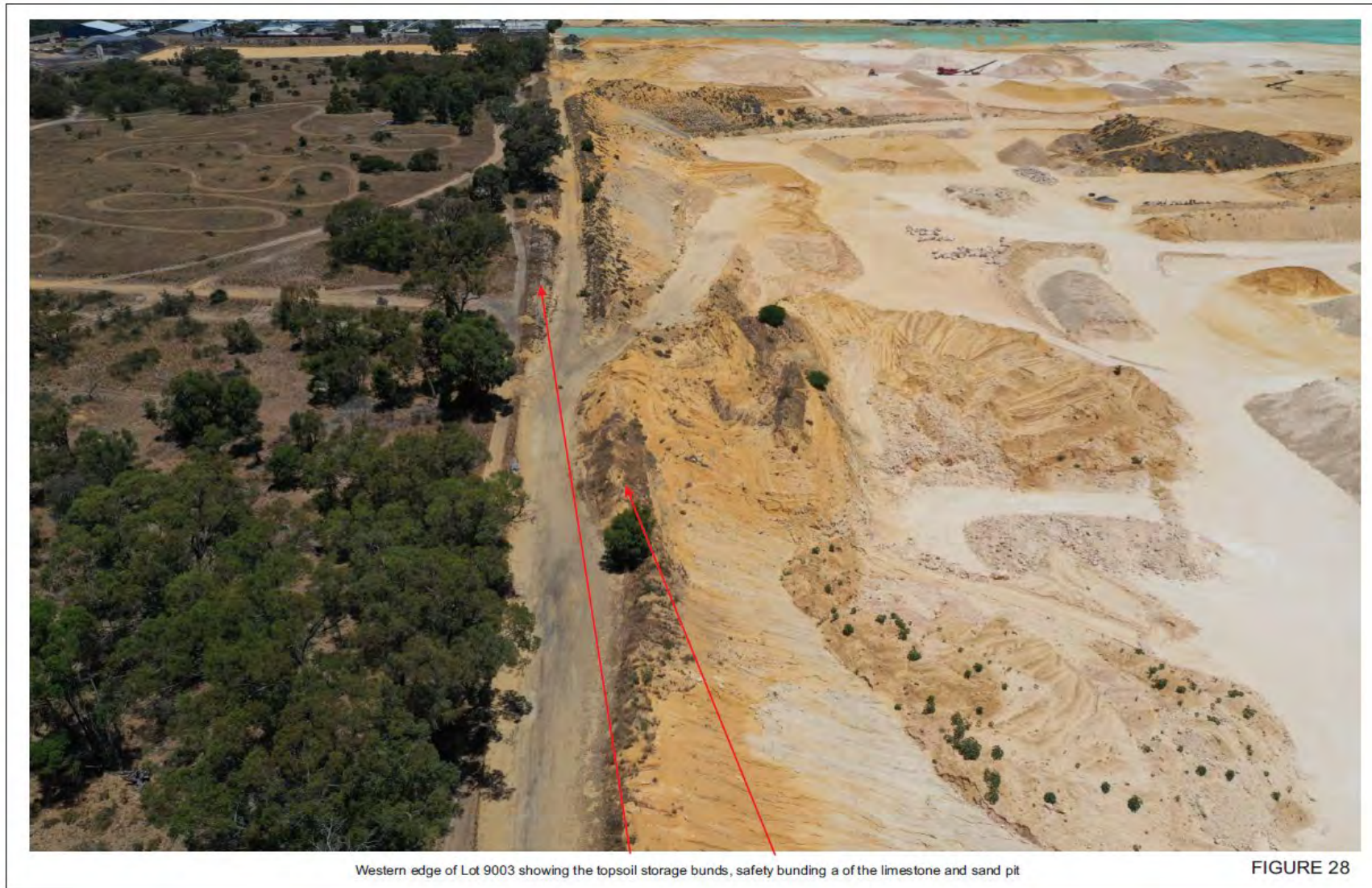
Figure 28: Western edge of Lot 9003 showing topsoil storage bunds and a bund of limestone
