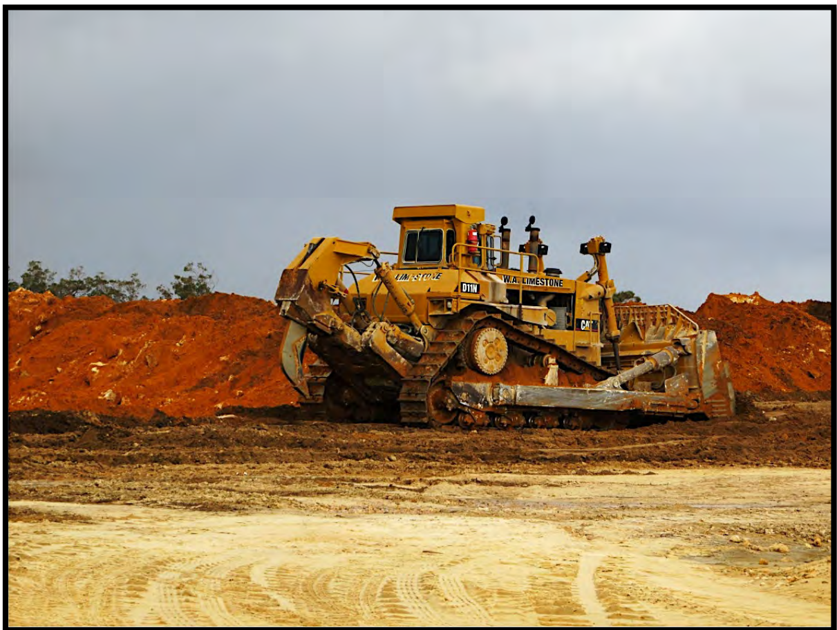
Figure 6: Bulldozer working in limestone
