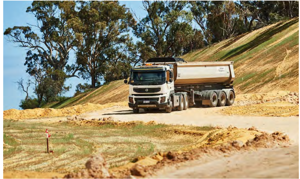
Example of a completed stabilised sand surface
