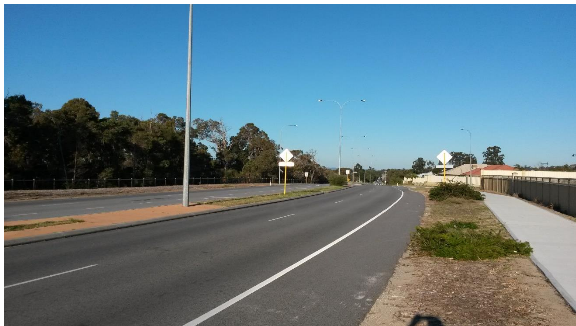
Figure 5: Eastbound view along Caporn Street from Pinjar Road intersection
