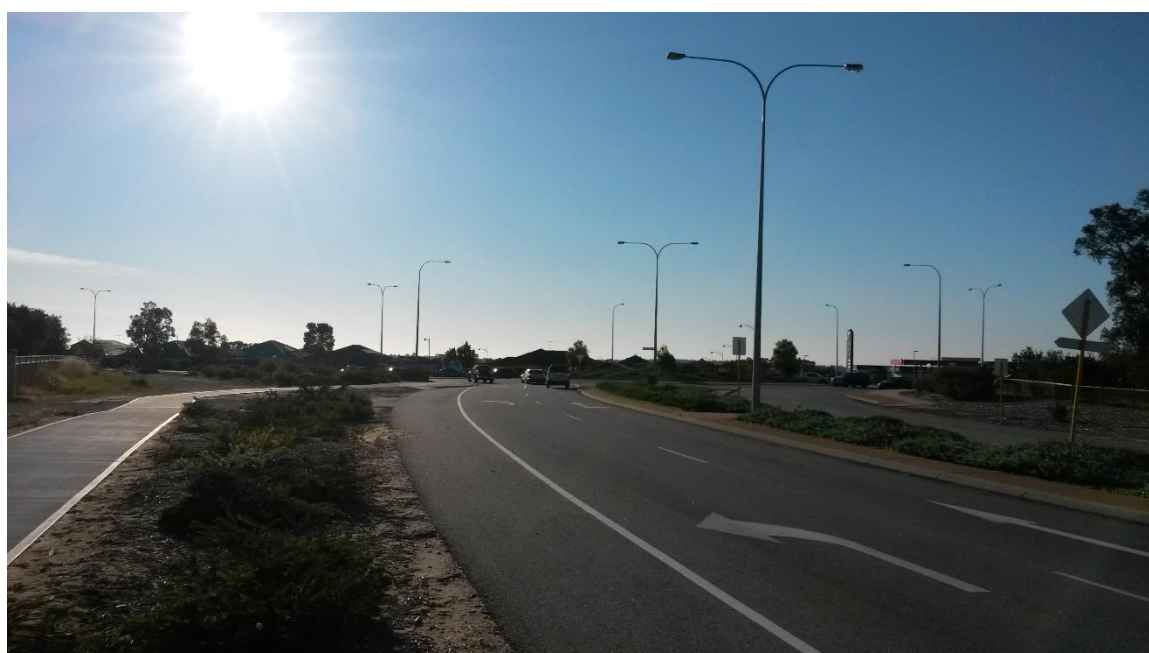
Figure 6: Westbound view along Caporn Street towards Pinjar Road intersection
