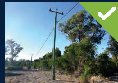
Compliant: cleared buffer zone around power poles
