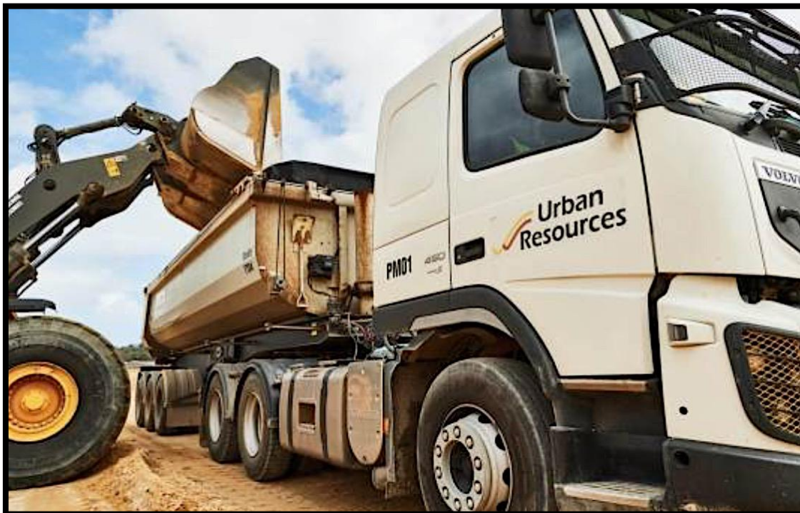
Figure 8: Loading sand onto road truck
