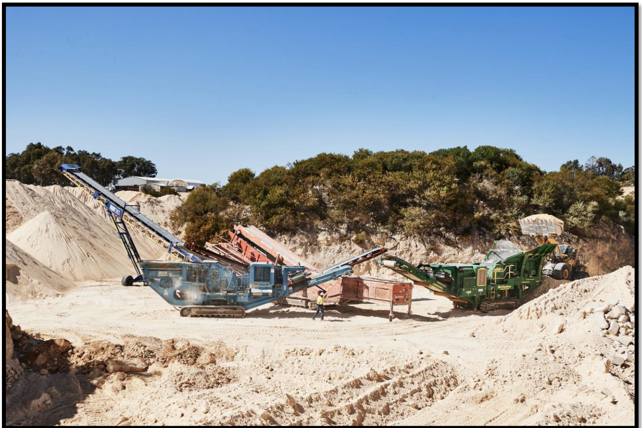
Figure 10: Crushing plant located on the floor of a limestone pit
