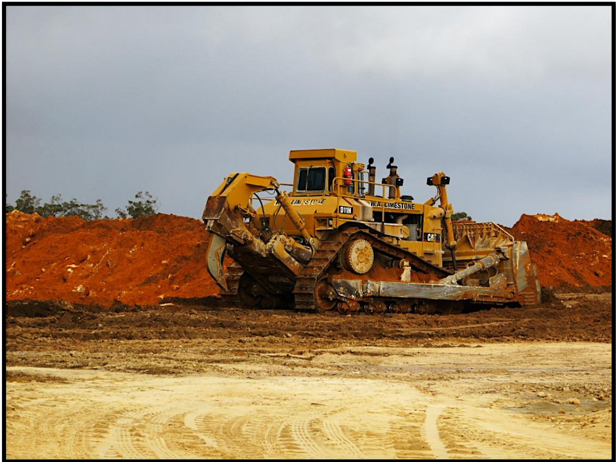
Figure 6: Bulldozer working in limestone
