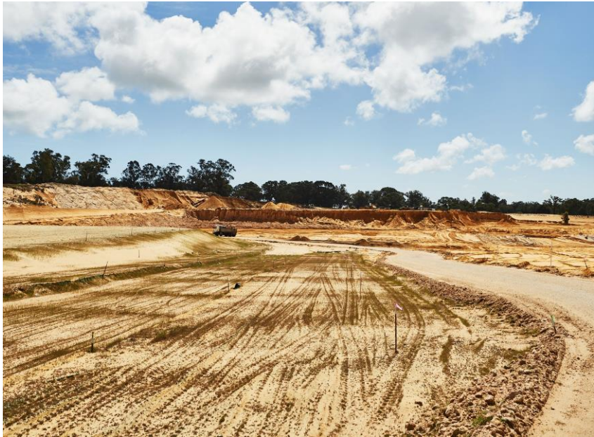
Typical excavation with a completed floor
