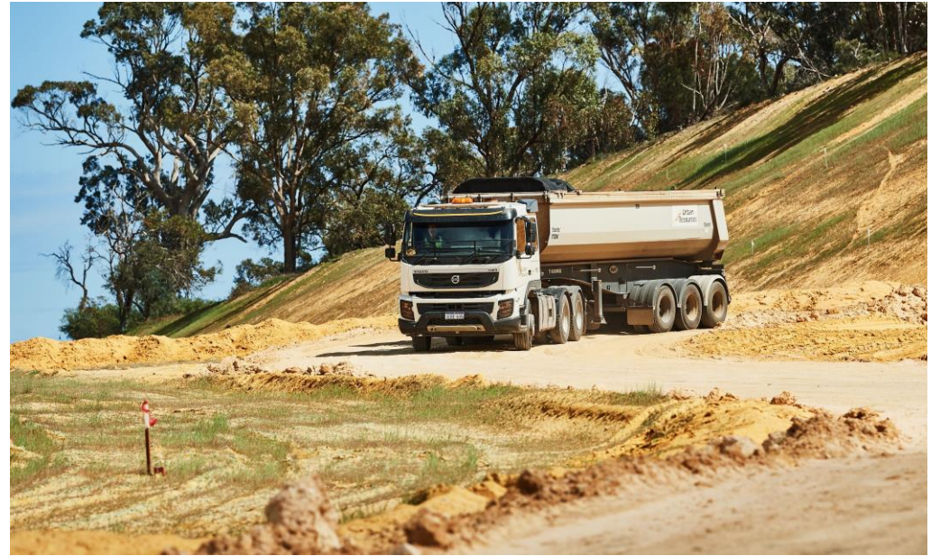
Example of a completed stabilised sand surface
