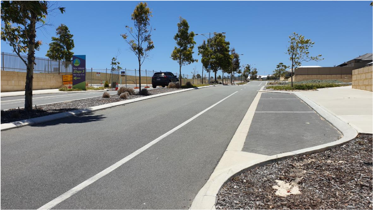
Figure 6: Intersection of Spinnaker Boulevard / Castlemead Drive
