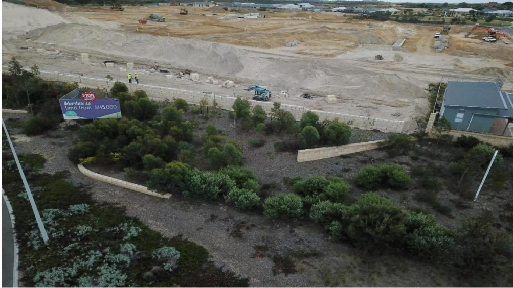
Figure 1: Evidence of civil engineering and other works progressing at Stage 3 Vertex
