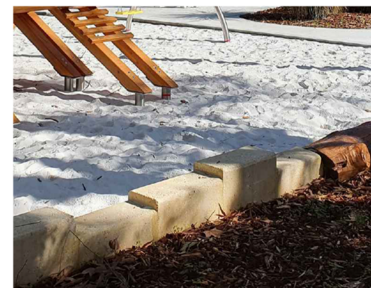
LIMESTONE EDGE TYPE 2 - STEPPED AND LANDSCAPE ROCKS TO CREATE ADDITIONAL PLAY VALUE
